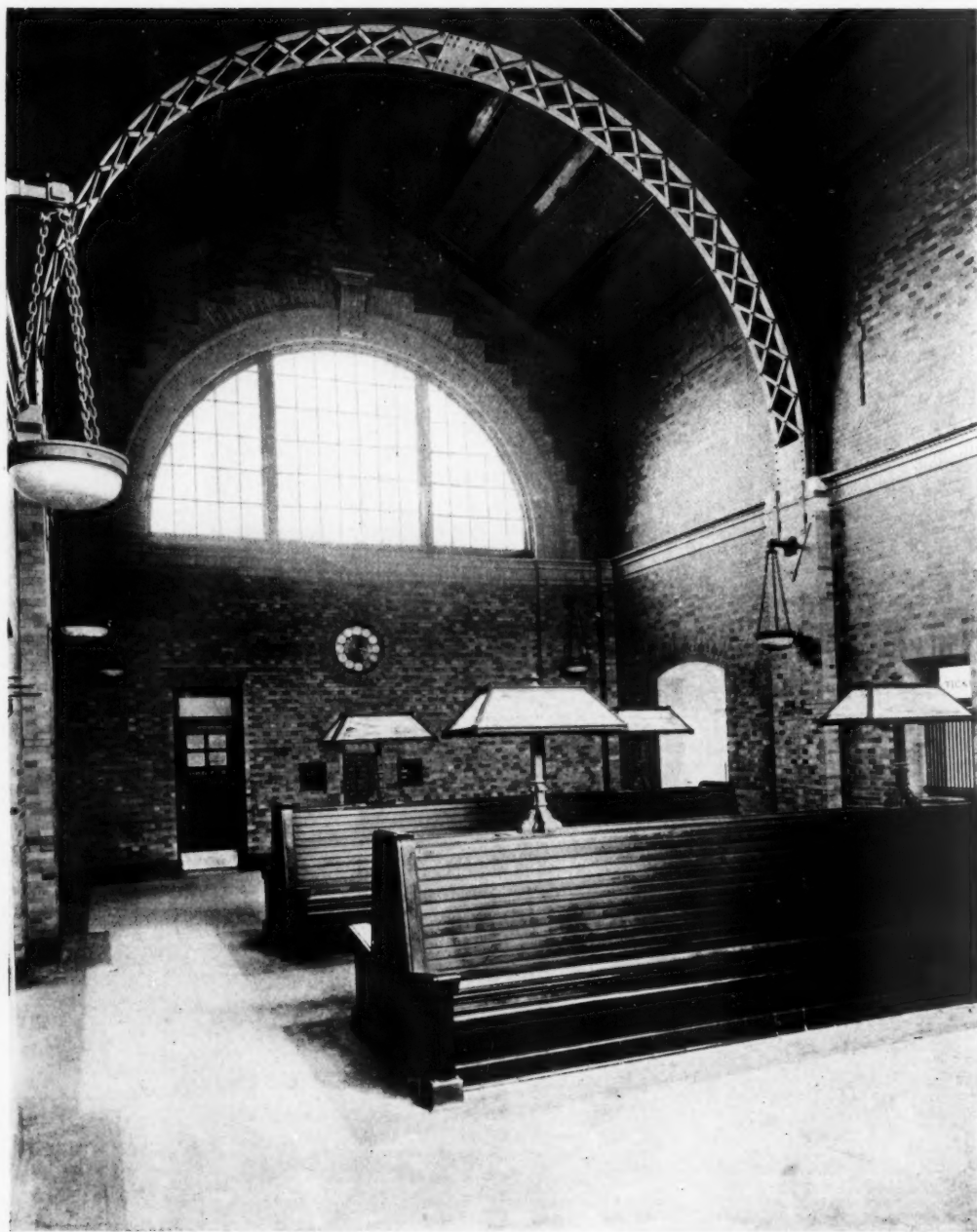
WAITING ROOM, MONTCLAIR STATION, D., L. & W. R. R.
