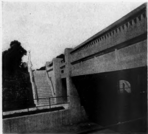
BRIDGE OVER STREET, WATSESSING.
