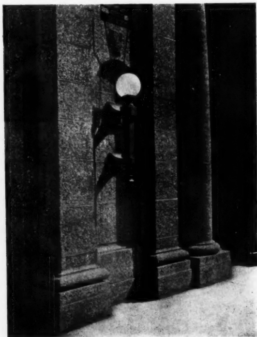
DETAIL, SHOWING SURFACE TEXTURE, MONTCLAIR STATION
