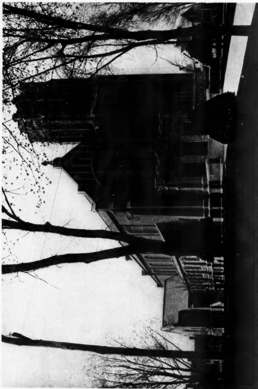
The building is built of cherry red brick with white mortar joints, grey terra cotta trimmings and unfading green slate roof. The interior finish is brown ash and it has a semi-indirect electric lighting and low pressure steam heating and a gravity system of ventilation.
