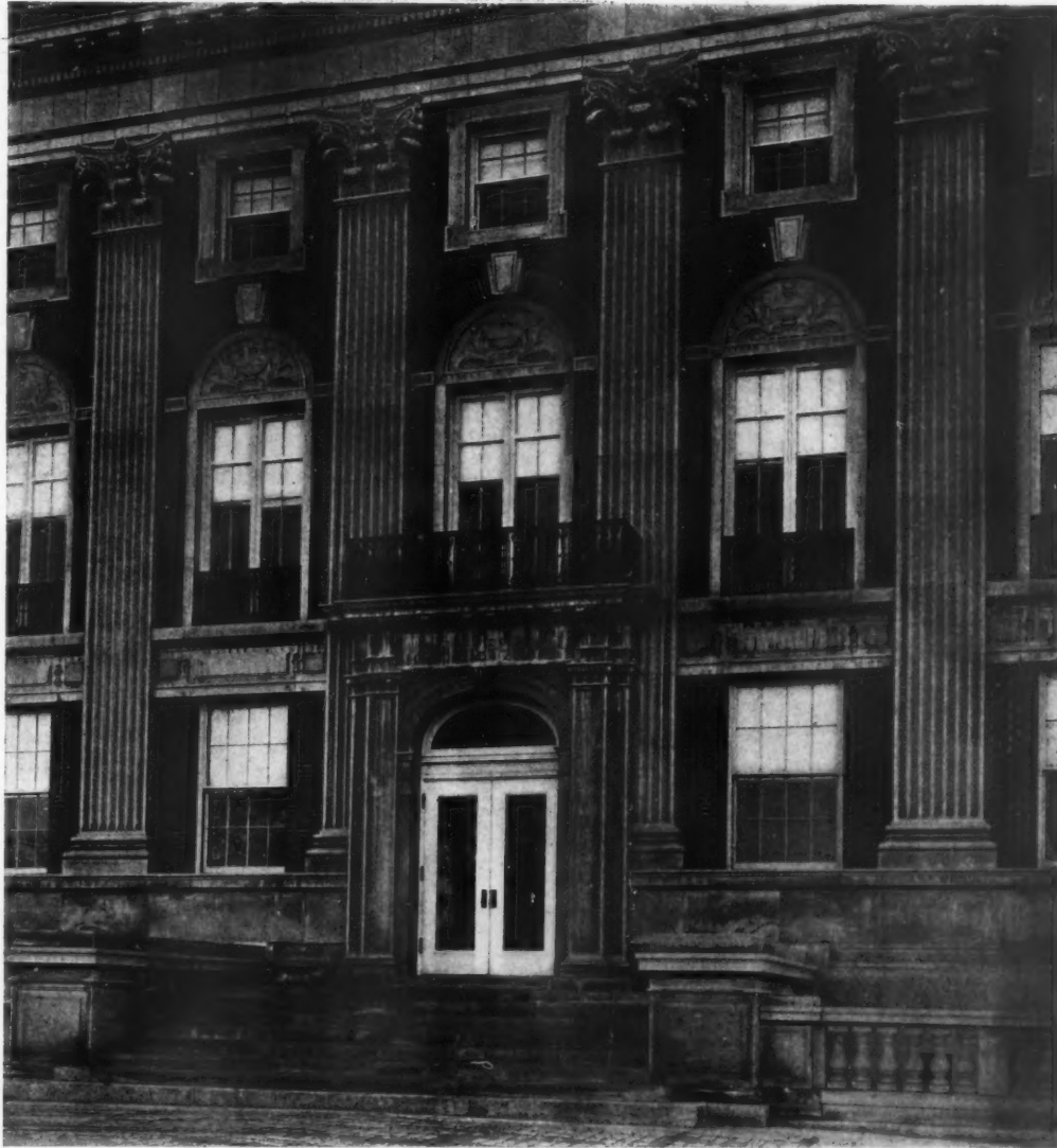
DETAIL OF ADMINISTRATION BUILDING FACADE
