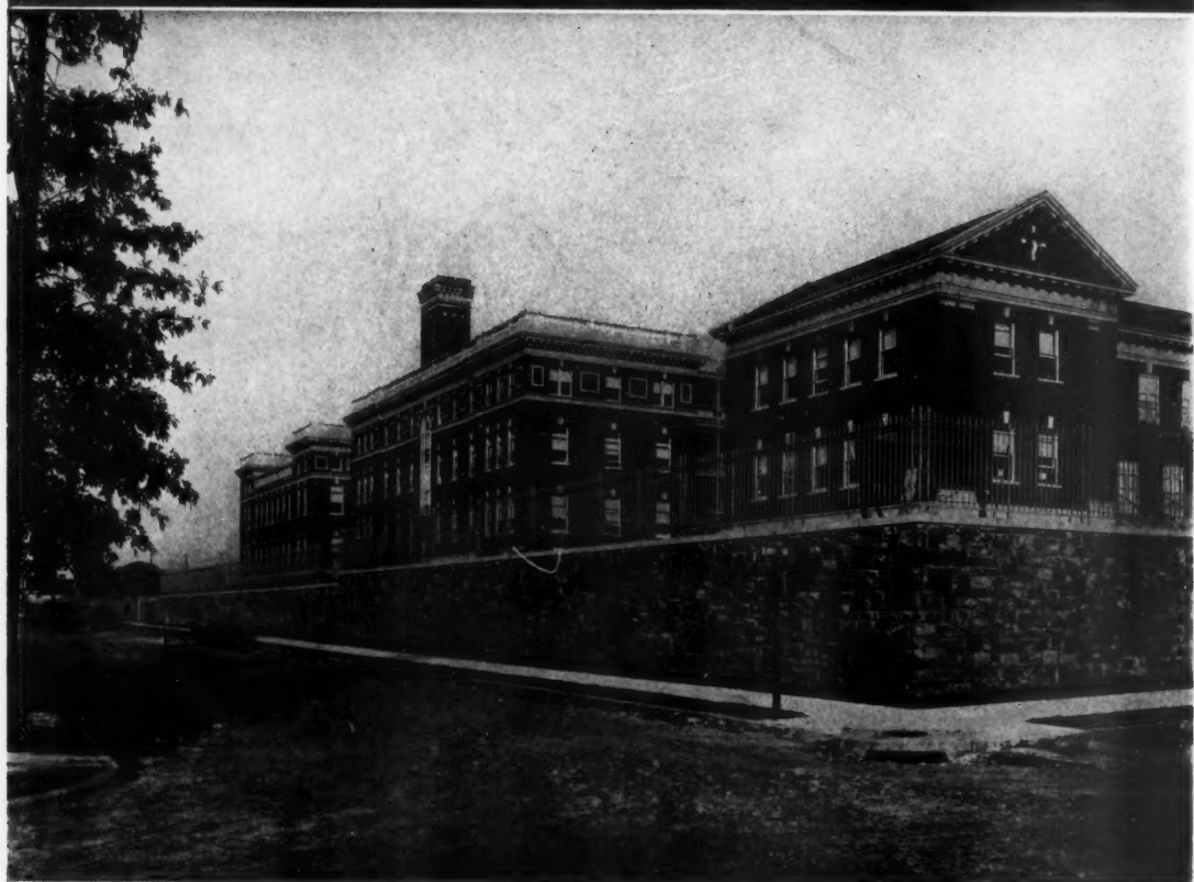
ABOVE, VIEW OF EASTERLY HALF OF SOUTH SIDE; BELOW, VIEW OF WEST SIDE
