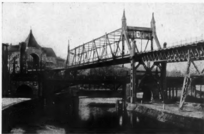
A NOVEL EXPEDIENT ON THE ELEVATED RAILWAY IN BERLIN The elevated structure, after passing through a building, bridges the Landwehr Canal over the Anhalter Railroad Bridge. The canal, street, railroad bridge and elevated bridge were built successively as the city developed.
