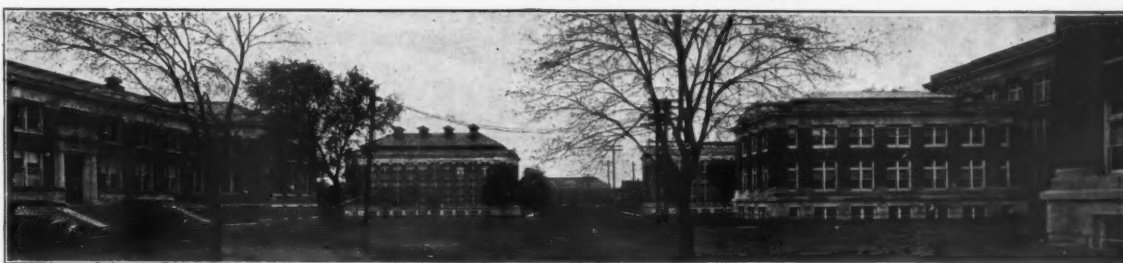
Experimental Laboratory and Main Engineering Building, University of Minnesota. Architect, Clarence H. Johnson. Best Bros. Keene's Cement Used.
