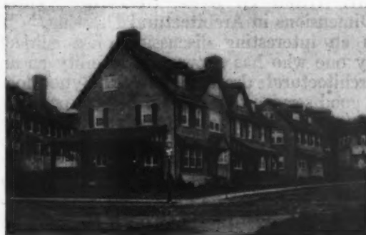
“QUADRUPLE” HOUSE, CHESTNUT HILL, PA. MESSRS. DUHRING, OKIE & ZIEGLER, ARCHITECTS
