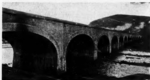
CONCRETE BRIDGE ON B. & O. R. R., CUMBERLAND, MD.
