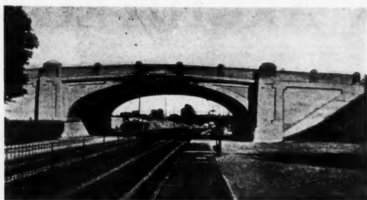
"BALA" BRIDGE ON SCHUYLKILL DIVISION, PENNSYLVANIA RAILROAD
