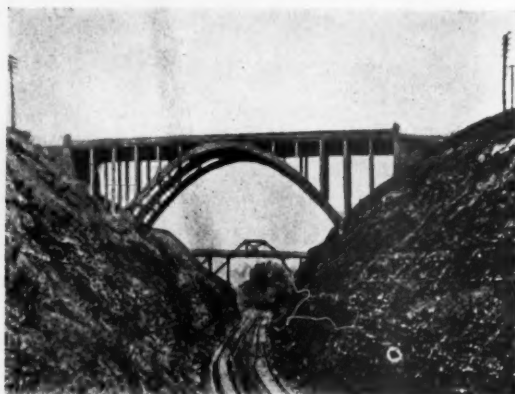
BRIDGE AT ELLSWORTH, PA., SHOWING AWKWARD APPEARANCE OF PARABOLIC ARCH
