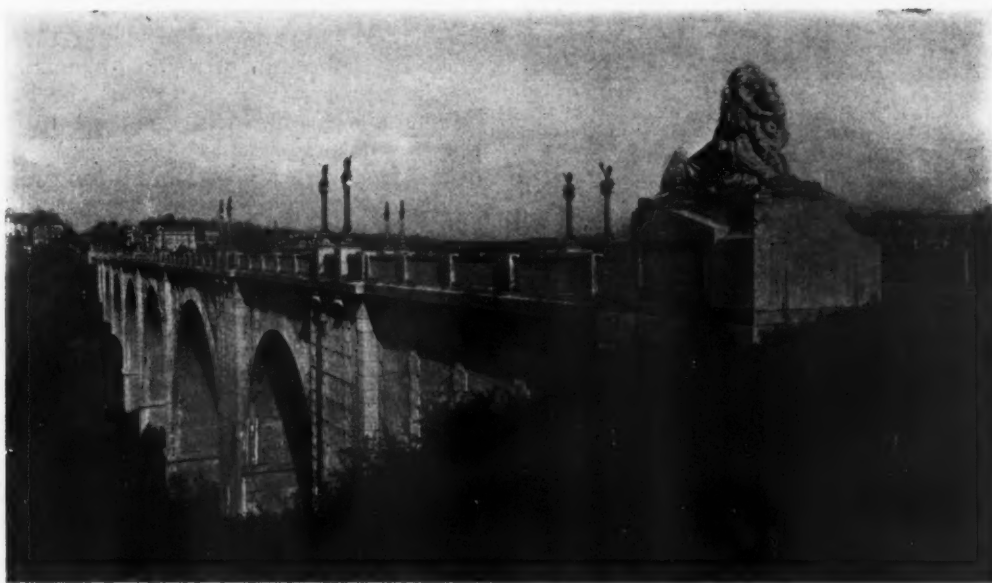
CONNECTICUT AVENUE BRIDGE, WASHINGTON, D. C. EDWARD PEARCE CASEY, ARCHITECT
