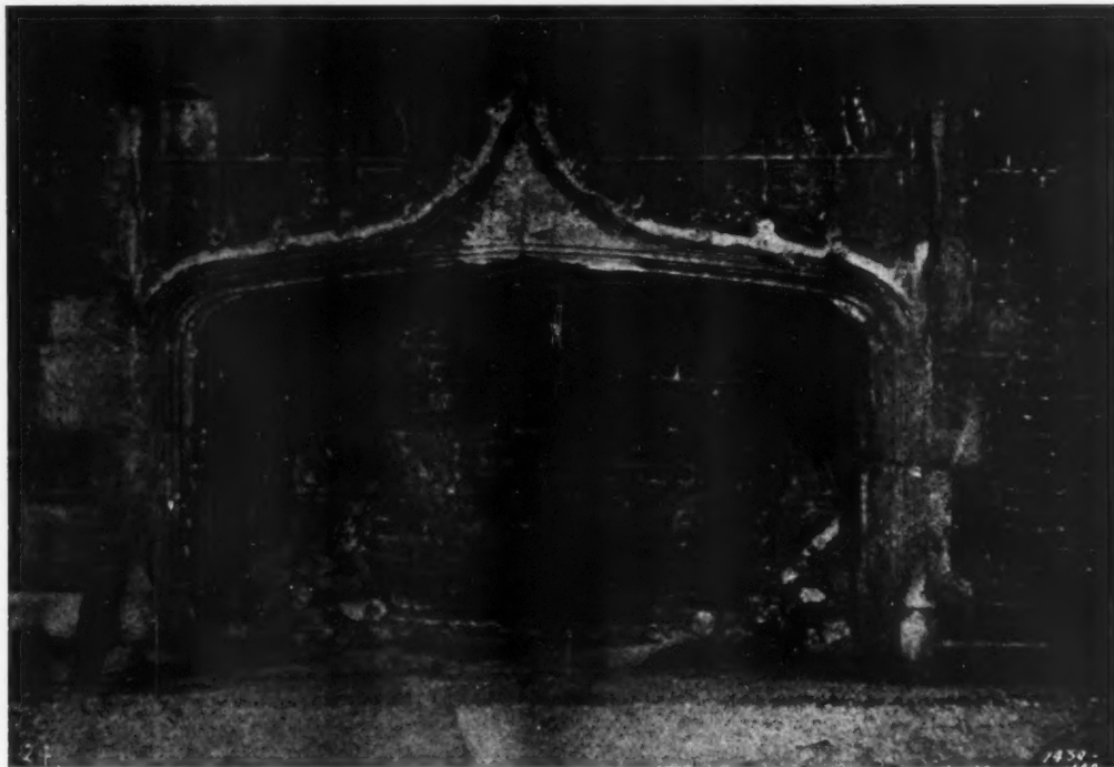
FIG. 1.—CHIMNEY PIECE ON GROUND FLOOR, TATTERSHALL CASTLE, LINCOLNSHIRE, ENGLAND
