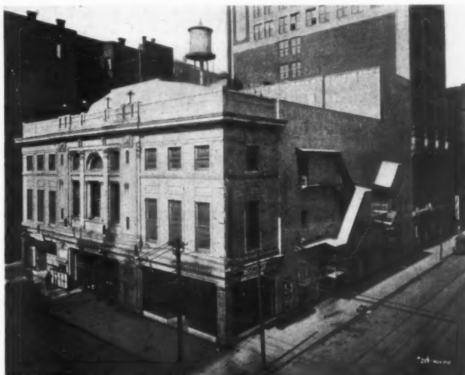
Kenyon Theatre Building, Pittsburgh N. Nirdlinger, Architect.
