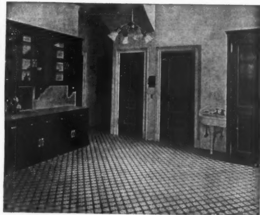
Kitchen—Horton Residence, Middletown, N. Y.
