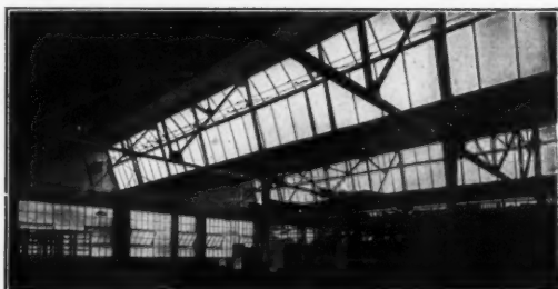
Pond Continuous Sash in Sawtooths. Lupton Steel Sash in Side Walls.
