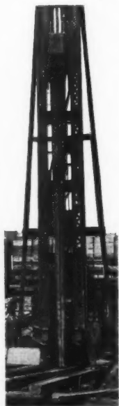
This shows the mandrel which receives the blow of the hammer, saving the shell from injury.
