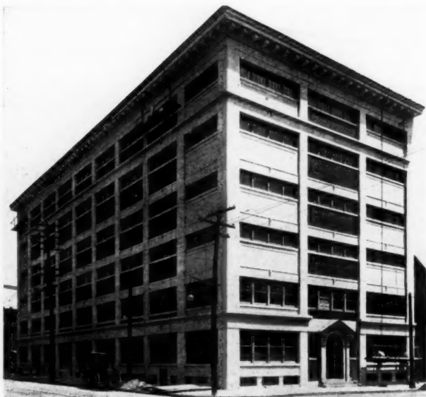
TURNER Construction Co. 11 Broadway, New York City
