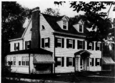
Residence, Cranford, N. J., Oakley & Sons, Architects. Floors soundproofed with Hydrex-Saniflor.
