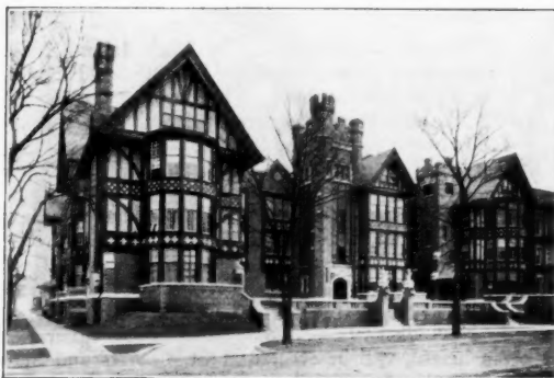
The Gables, Chicago J. E. O. Pridmore, Architect Kewanee Garbage Burner and Boiler Installed
