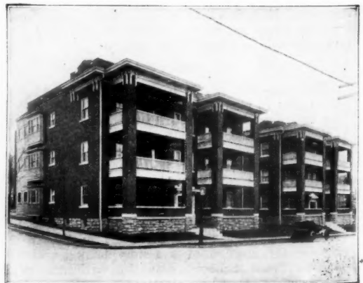
Shryock Apartments, Kansas City Thurtle-Thayer Co., Architects Kewanee Garbage Burner and Boiler Installed
