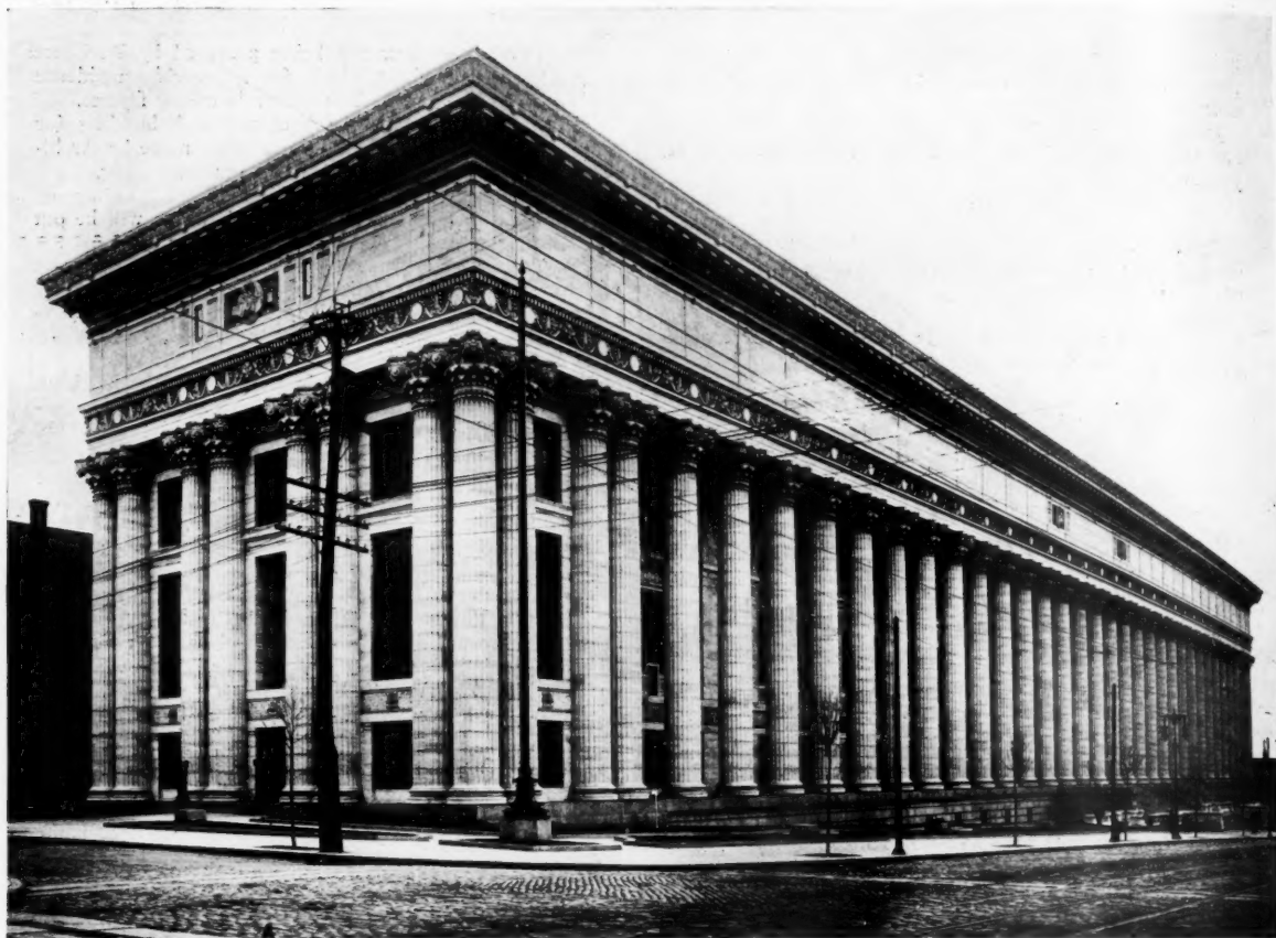
State Education Building, Albany, N. Y.
