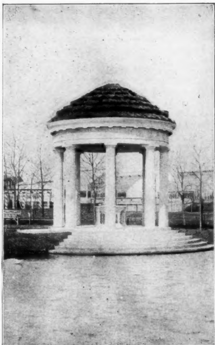
PAVILION OF NEWMAN ERB, ELBERON, N. J. Clarence Luce, Architect. J. C. Kraus, Contractor
