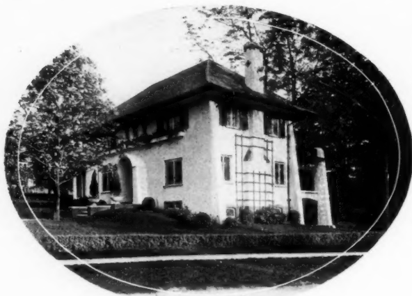
Residence, W. P. PLUMMER Douglaston, Long Island
