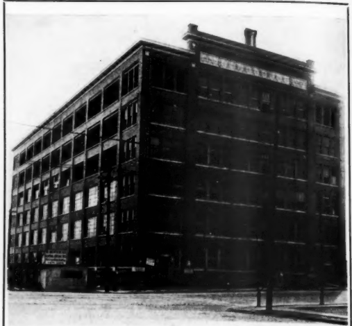
BUILDING FOR SCHORSCH & COMPANY, BOROUGH OF BRONX, NEW YORK C. B. COMSTOCK, Architect
