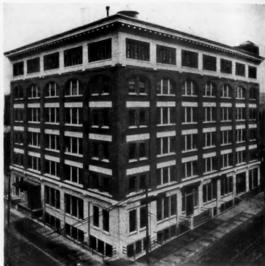
Howard Chapman, Architect.
