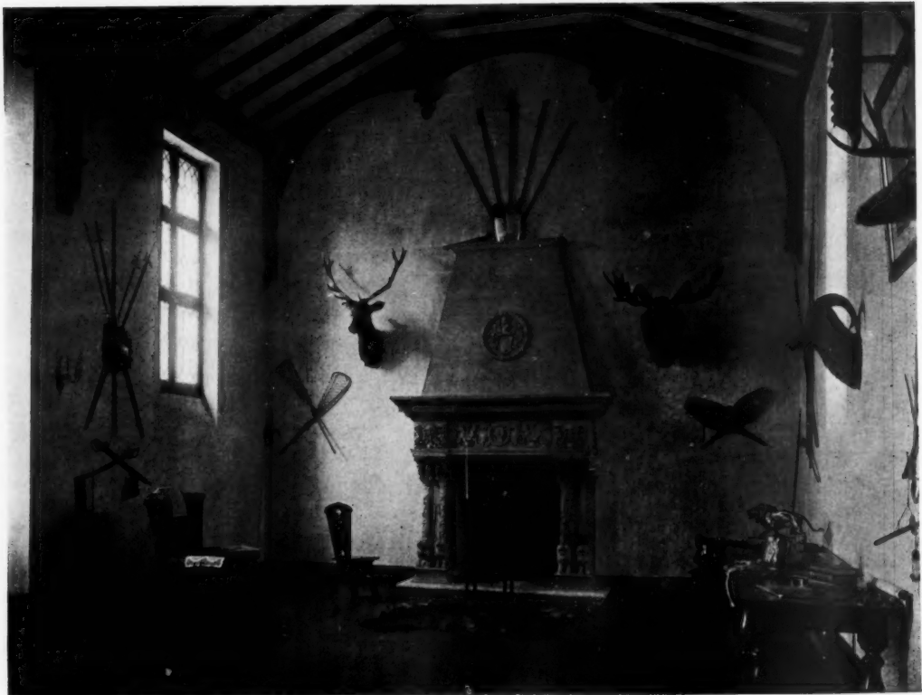
MAIN ENTRANCE AND END OF GREAT HALL
