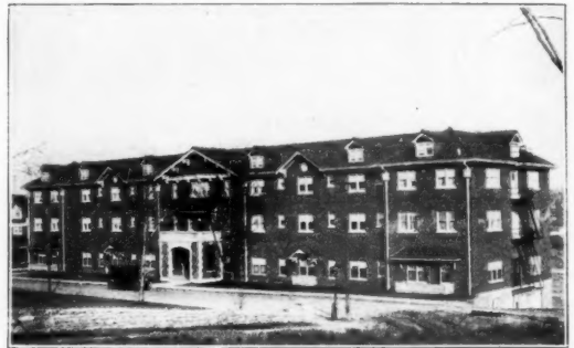
Rockhill Manor, Kansas City Roger Gilman, Architect Kewanee Garbage Burner and Boiler Installed
