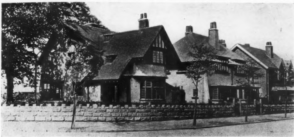
COTTAGES AT BOURNEVILLE
