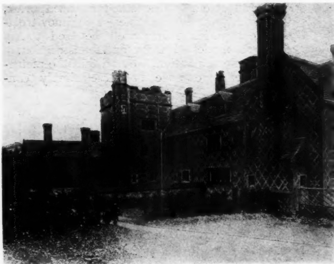
SHIPLAKE COURT, HENLEY-ON-THAMES, ENGLAND MESSRS. GEORGE & PITE, ARCHITECTS
