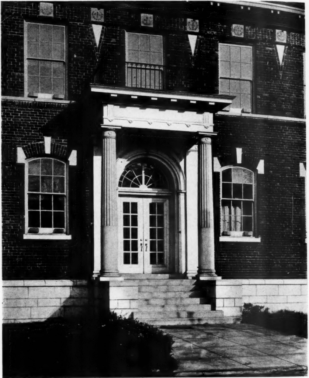
DETAIL OF MAIN ENTRANCE
