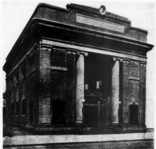
WEST HUDSON COUNTY TRUST CO., HARRISON, N. J. MESSRS. CROW, LEWIS & WICKENHOEFER, ARCHITECTS
