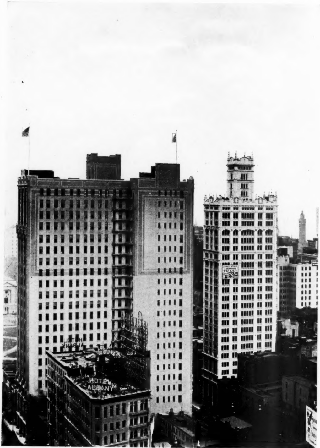
At Left ,—LEWISOHN BUILDING, EXTENDING THROUGH FROM FORTIETH TO THIRTY-NINTH STREET
