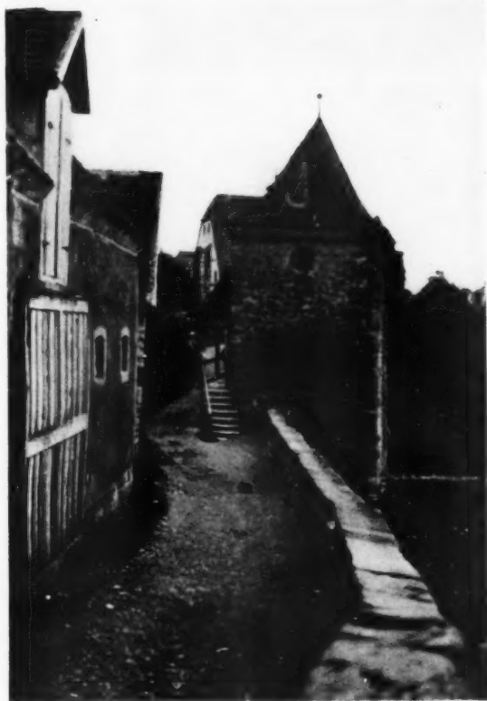
LOOKING ALONG TOWN WALL
