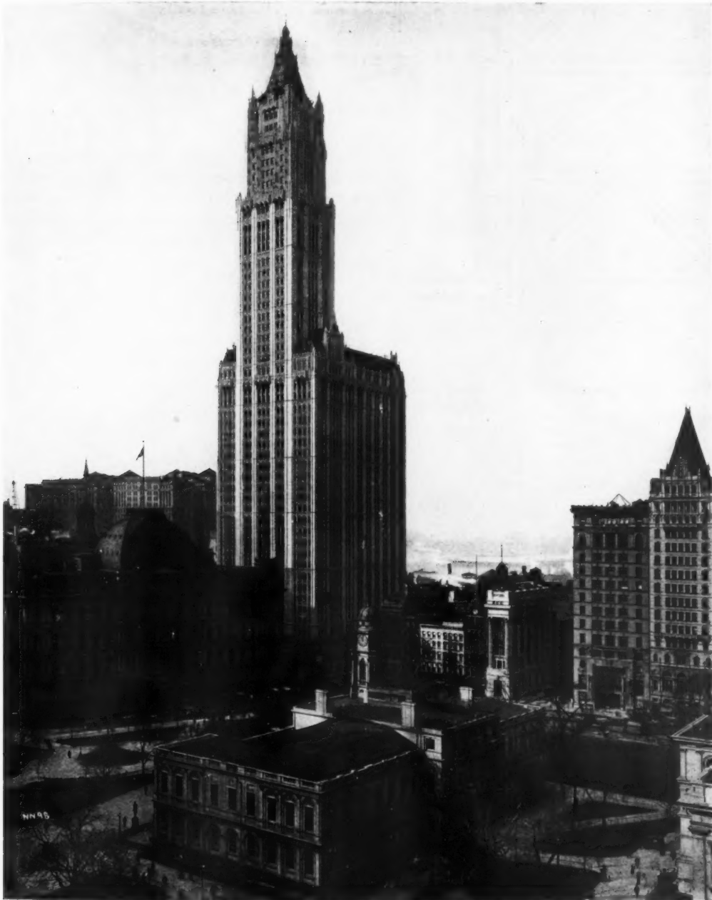
VIEW LOOKING SOUTHWEST, CITY HALL IN FOREGROUND
