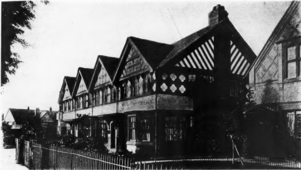
COTTAGES AT PORT SUNLIGHT
