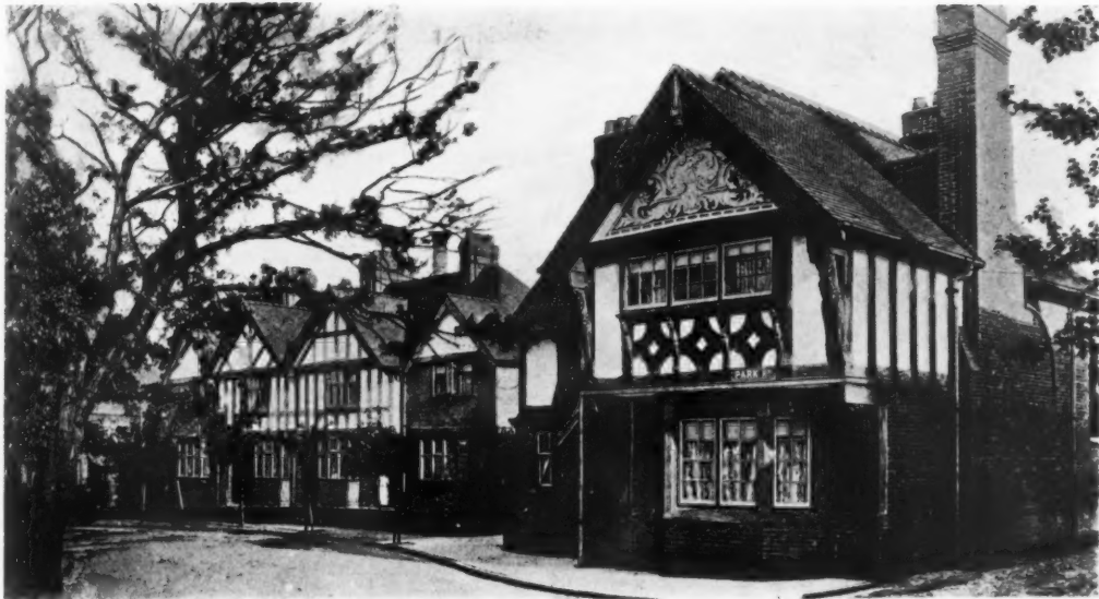
COTTAGES AT PORT SUNLIGHT
