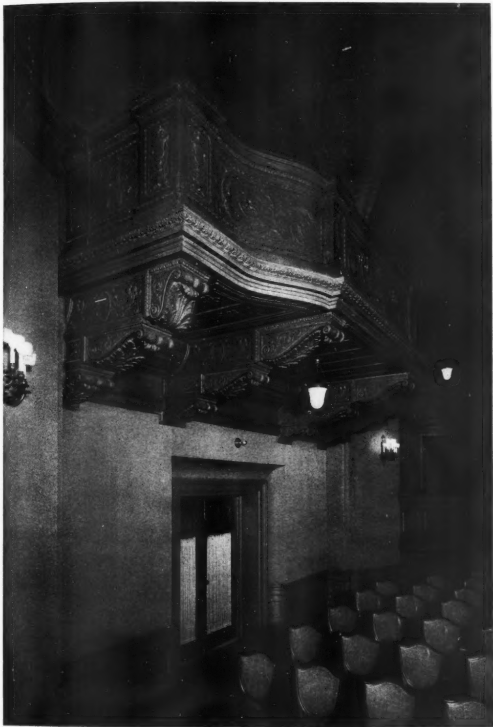
DETAIL OF BALCONY IN ASSEMBLY ROOM
