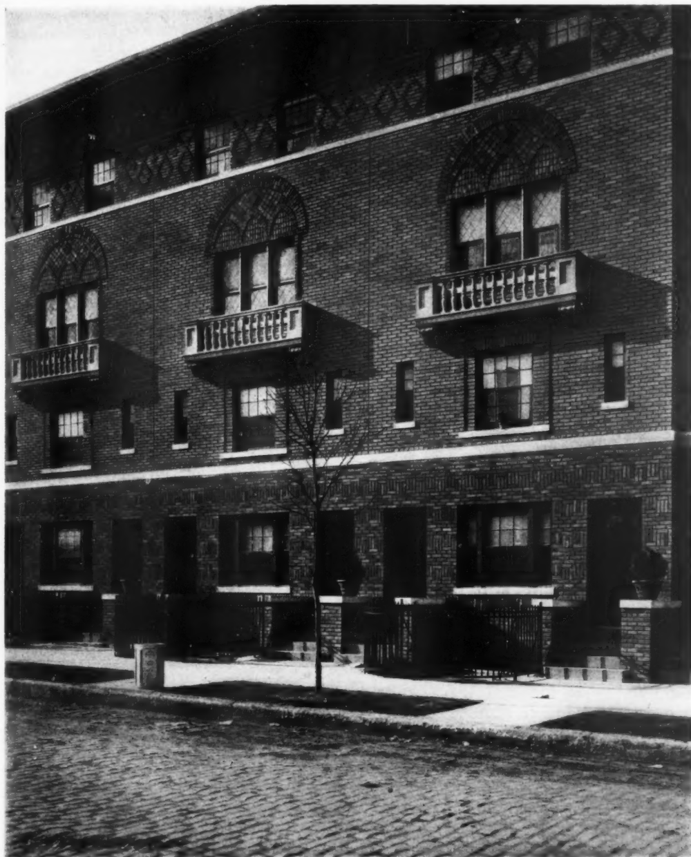
DETAIL OF A ROW OF HOUSES IN BROOKLYN, N. Y.
