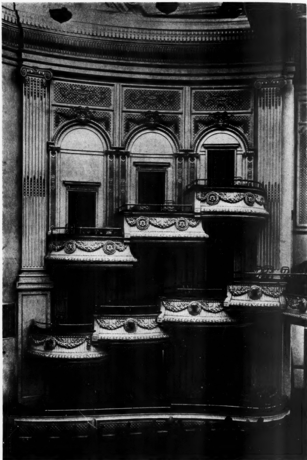
DETAIL OF BOXES
