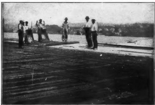
HY-RIB Concrete Roofs—Built without forms— Packard Motor Car Co., Detroit.
