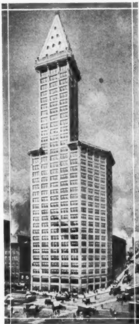
42-STORY L. C. SMITH BUILDING Seattle, Wash. GAGGIN & GAGGIN Architects The WHITNEY CO. Contractors
