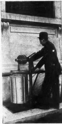
Hoist in Operation
