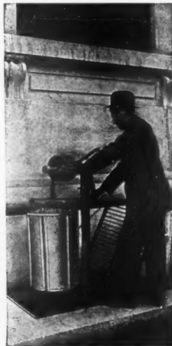
Hoist in Operation
