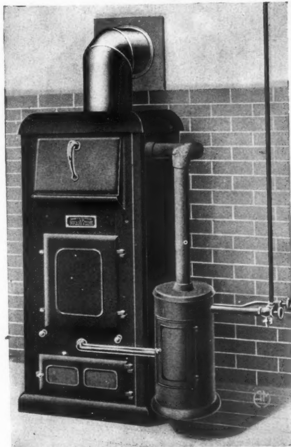
PYROFUSE TYPE M (Showing Gasoline Attachment)
