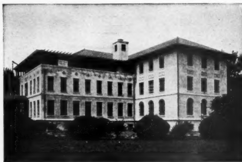
Special UNITED STEEL SASH in DETENTION BLDG. AND IMMIGRATION STATION, Gloucester, N. J. Ventilators are one light in height, extending full width of sash. Note at right that entire sash are pivoted at top and bottom.
