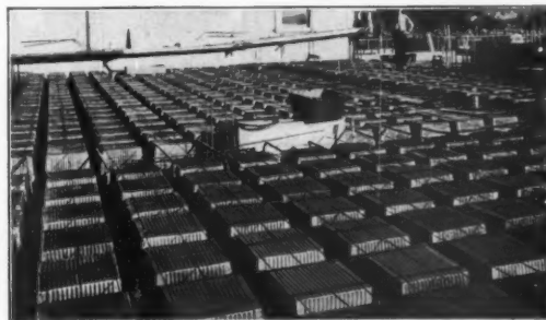
FLOREDOME Construction, Mt. Taber School, Portland, Ore. Note straight and true lines of FLOREDOMES and accurate spacing of joists.
