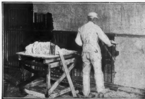
HY-RIB Partition—Note grounds for base-board and chair-rail.
