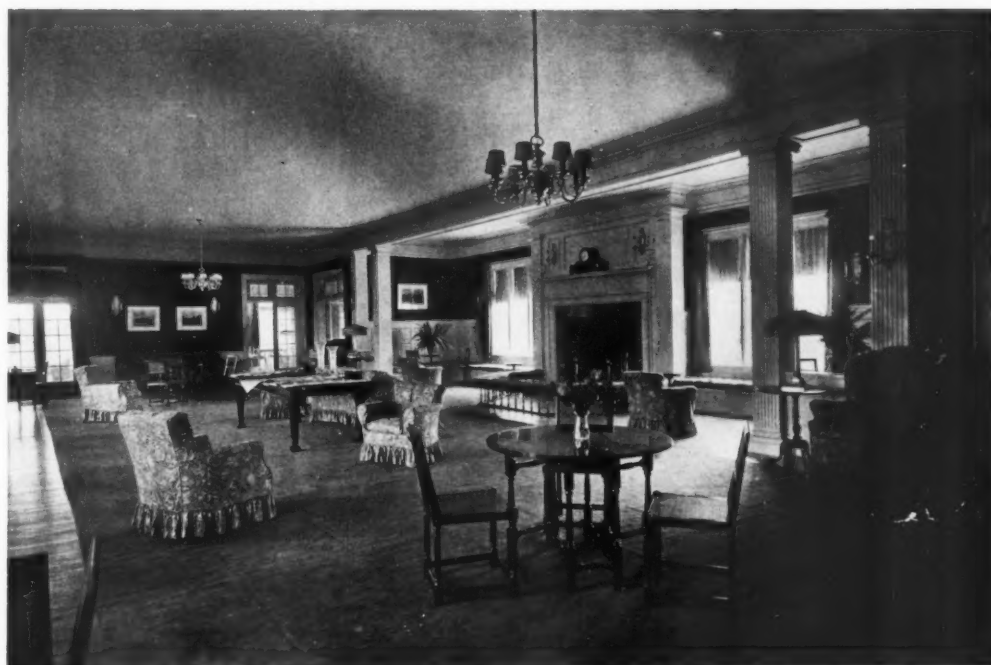
PIPING ROCK CLUB, LOCUST VALLEY, L. I., NEW YORK MR. GUY LOWELL, ARCHITECT
