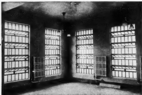
Special UNITED STEEL SASH in DETENTION BLDG. AND IMMIGRATION STATION, Gloucester, N. J. Ventilators are one light in height, extending full width of sash. Note at right that entire sash are pivoted at top and bottom.
