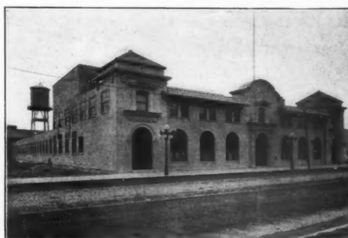
Artistic HY-RIB Concrete Sidings—Built without forms— Sunset Publishing Co., San Francisco, Cal.
