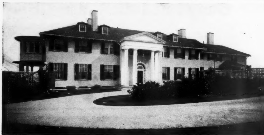
Residence of J. A. Burnham, Wenham, Mass. Winslow & Bigelow, Architects. NEPONSET Waterproof Building Paper Used.
