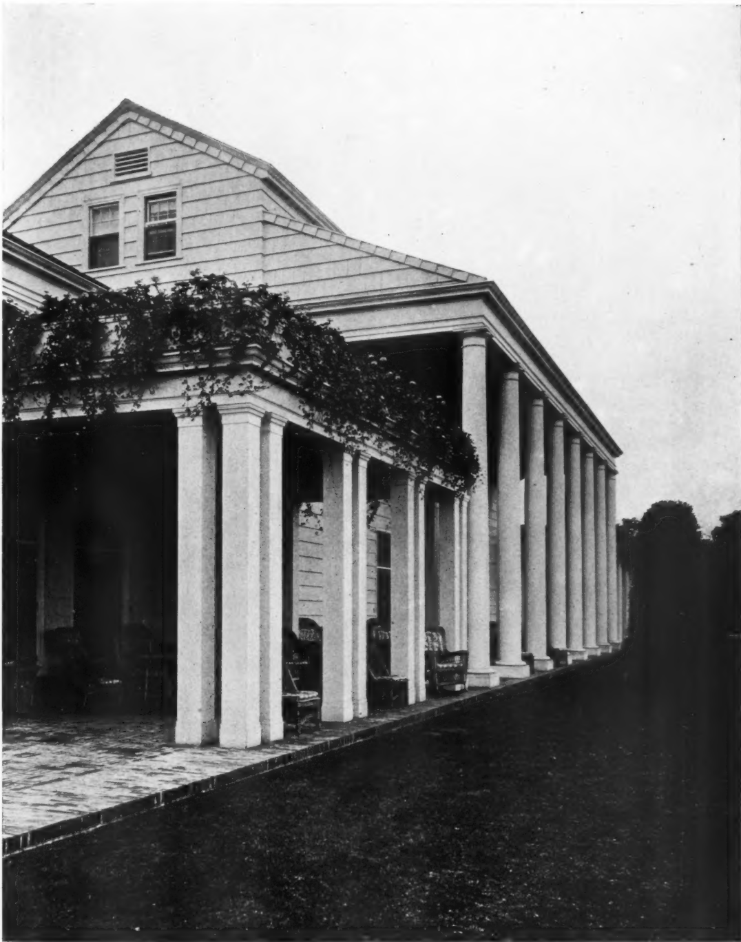
PIPING ROCK CLUB, LOCUST VALLEY, L. I., NEW YORK MR. GUY LOWELL, ARCHITECT
