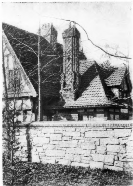
A GATE LODGE AT GREAT NECK, L. I., N. Y. MR. JOHN RUSSELL POPE, ARCHITECT
