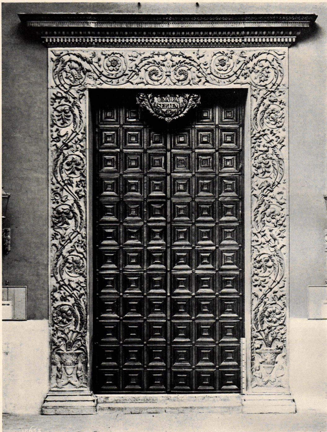
DETAIL OF PRINCIPAL ENTRANCE
