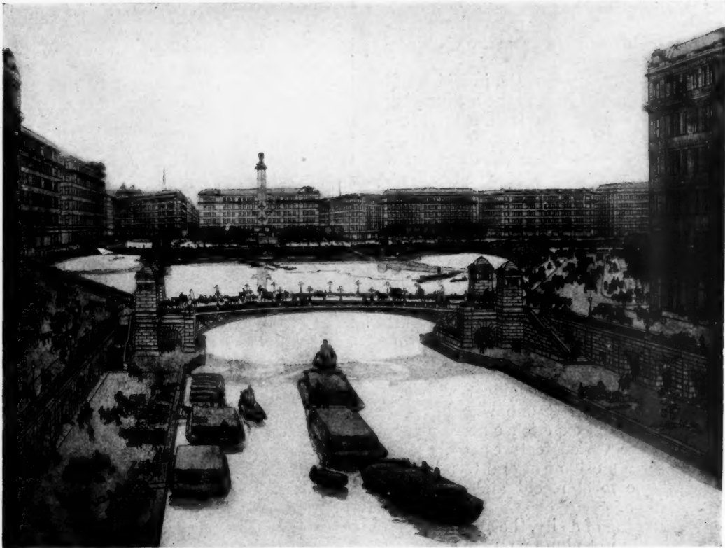
PROPOSED REARRANGEMENT OF STREETS AND WATERWAYS, CHICAGO, ILL. VIEW LOOKING NORTH ON THE SOUTH BRANCH OF THE CHICAGO RIVER, SHOWING METHOD OF HANDLING FREIGHT AND TRAFFIC ON DIFFERENT LEVELS. EXAMPLES OF A SIMILAR ARRANGEMENT EXIST AT DUSSELDORF, ALGIERS, BUDAPEST, GENEVA AND PARIS (Copyrighted by the Commercial Club)
