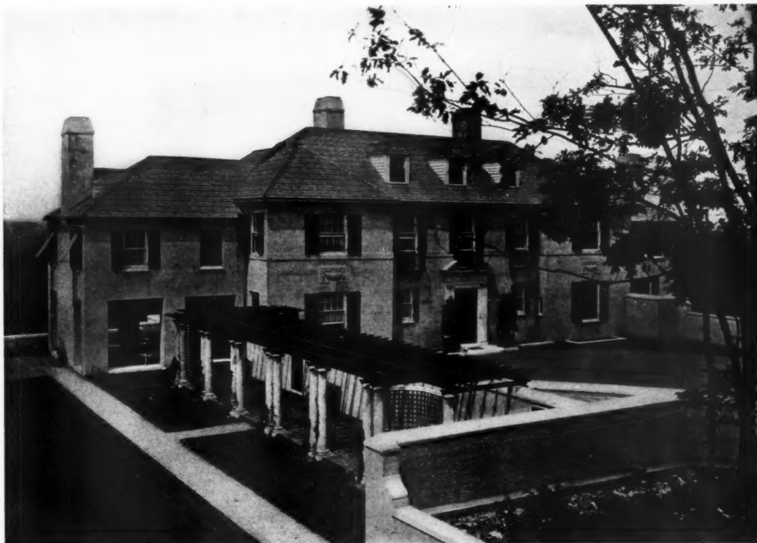
THE ENTRANCE COURT
