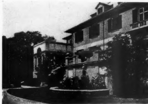
TERRACE OF A HOUSE AT BRYN MAWR, PA. MR. CHARLES A. PLATT, ARCHITECT
