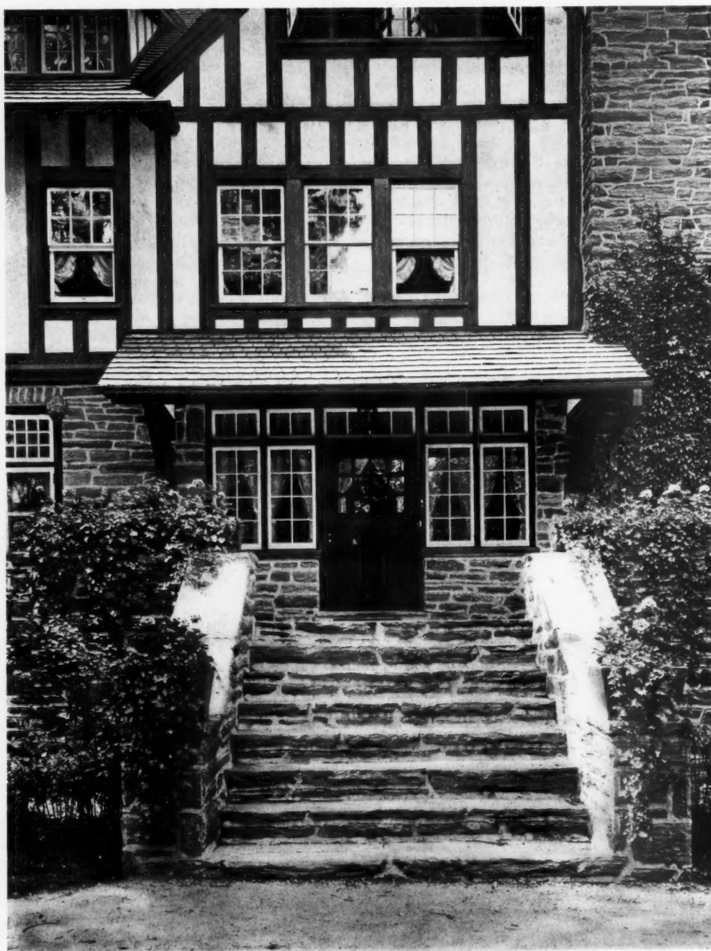
DETAIL OF ENTRANCE
