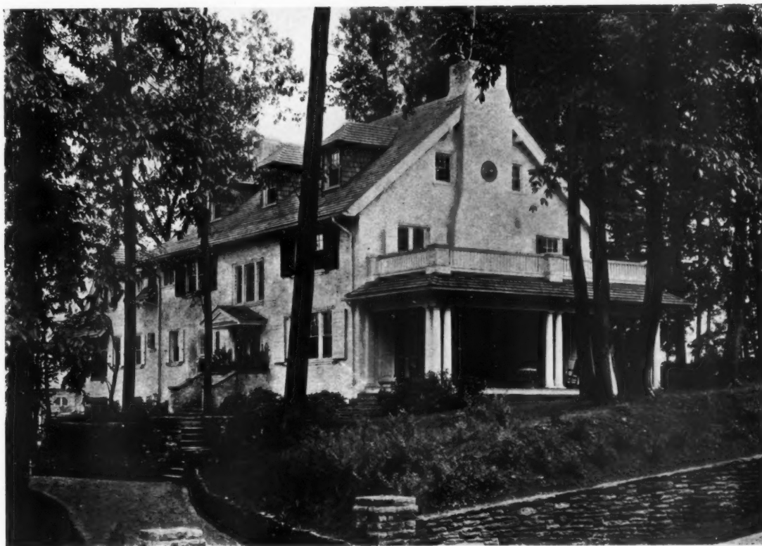
HOUSE OF FRANKLIN BAKER, JR., ESQ., GERMANTOWN, PHILADELPHIA. PA. MESSRS. DUHRING, OKIE & ZIEGLER, ARCHITECTS
