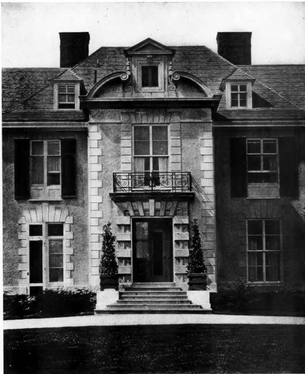
DETAIL OF ENTRANCE
