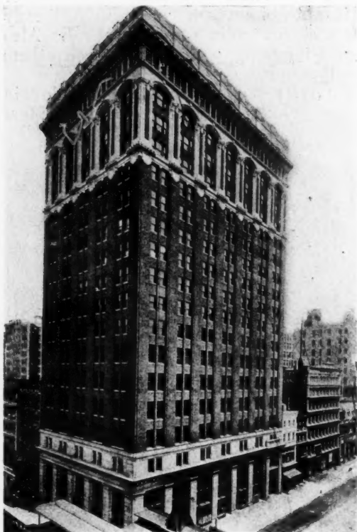
A LOFT BUILDING ON WEST 23d STREET, NEW YORK
