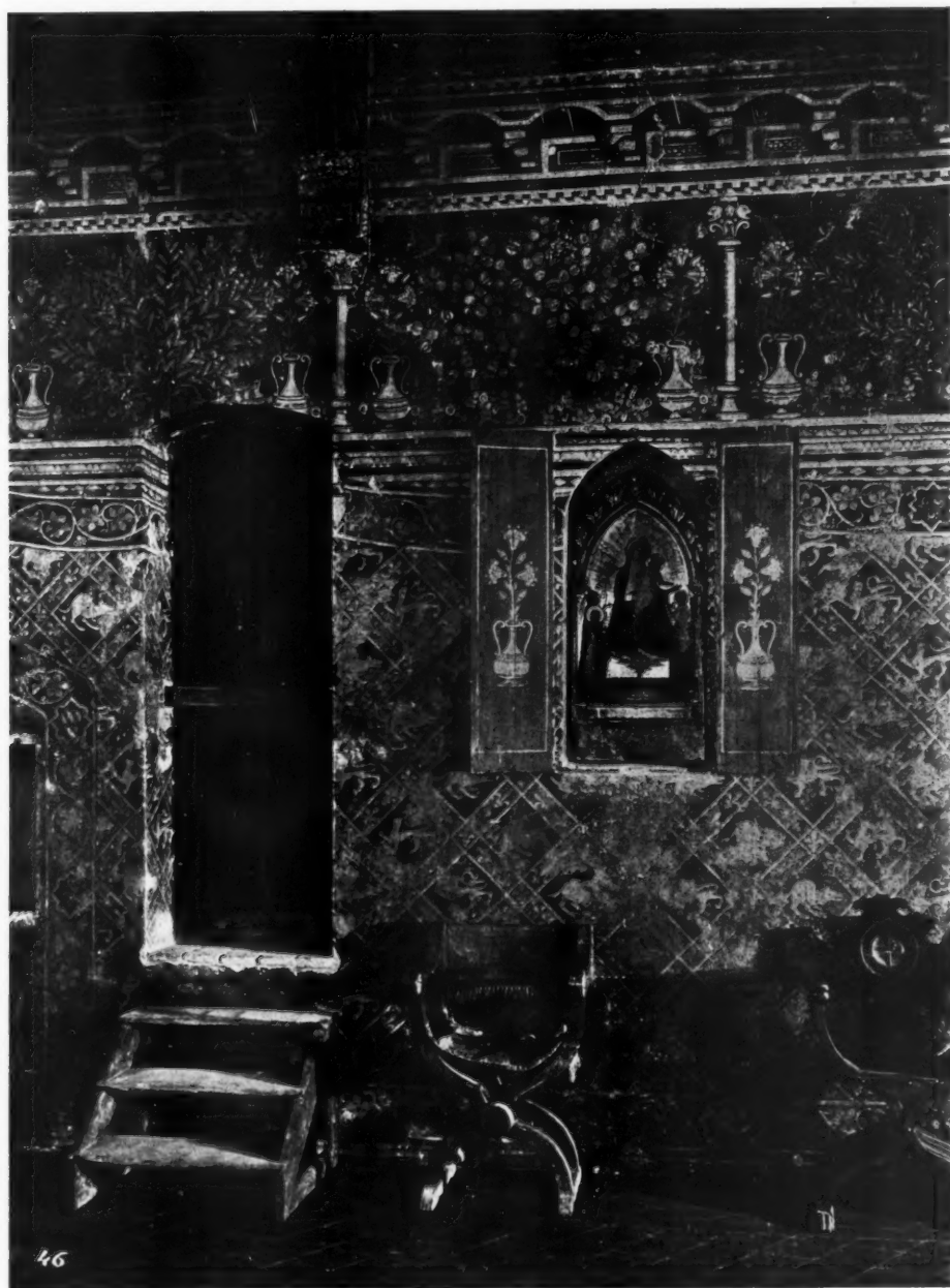
WALL DETAIL, SMALL APARTMENT ON THIRD FLOOR, SHOWING DECORATIVE MOTIVES
