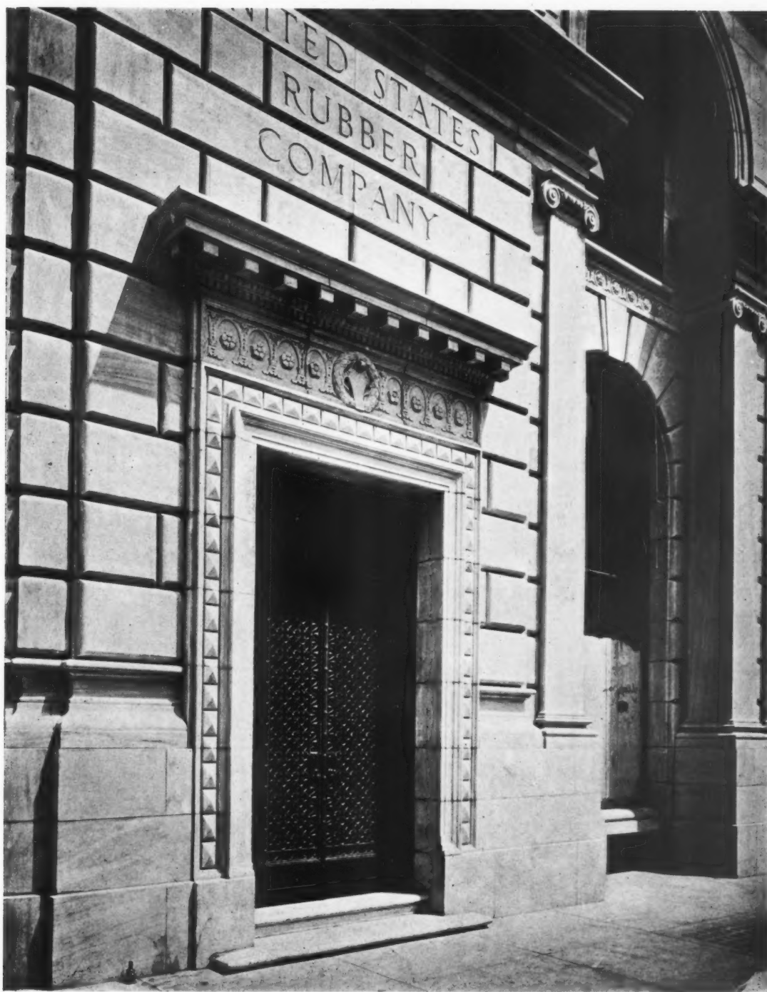
DETAIL OF AN ENTRANCE ON BROADWAY
