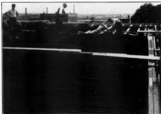
Hy-Rib with reinforced concrete beams. No centering required for slabs or beams, except board under beam and temporary joists under Hy-Rib.
