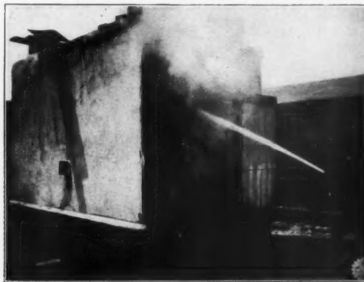
New York Fire Test on Hy-Rib Partitions. Subjected to a temperature of 1,700° Fahr. for one hour and then a stream of water at hydrant pressure.
