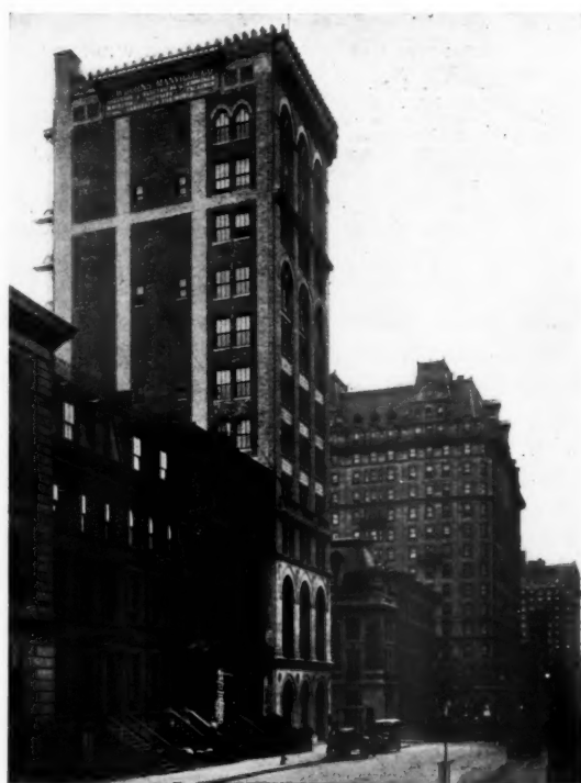
THE H. W. JOHNS-MANVILLE BUILDING
