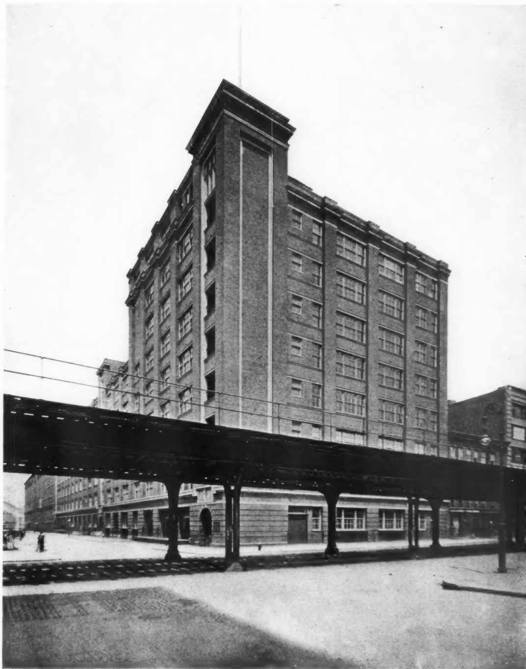
NEW YORK CITY BUILDING, NATIONAL BISCUIT COMPANY
