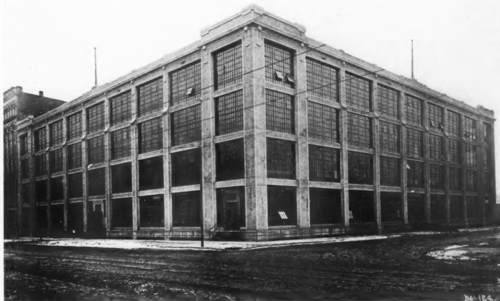
Above, MACHINE SHOP, PLANT OF MISSISSIPPI GLASS CO., ST. LOUIS, MO. Messrs. BRENECKE & FAY, Architects
