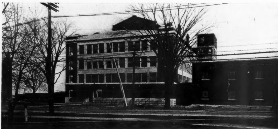
BUILDING FOR THE WOOLSON SPICE CO., TOLEDO, OHIO
