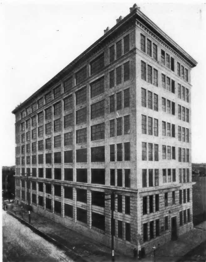
TURNER-CARTER CO. BUILDING, BROOKLYN, N. Y. Mr. FRANK J. HELME, Architect
