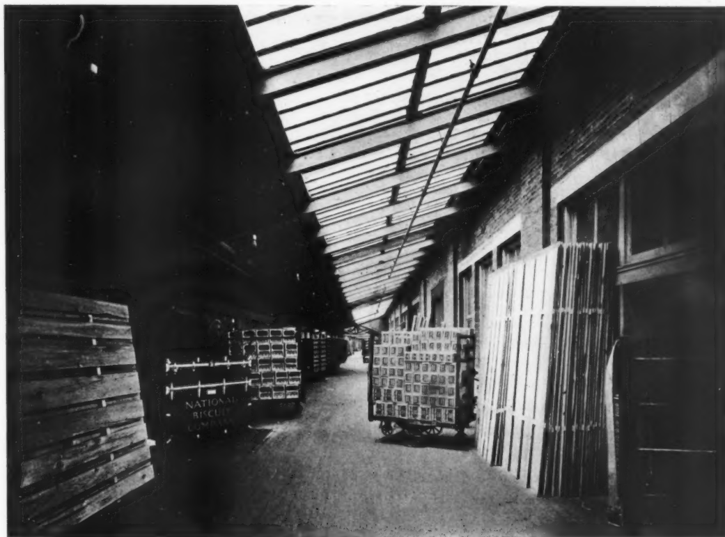
CAR LOADING PLATFORM NEW YORK BUILDING, NATIONAL BISCUIT CO. Mr. A. G. ZIMMERMAN, Architect
