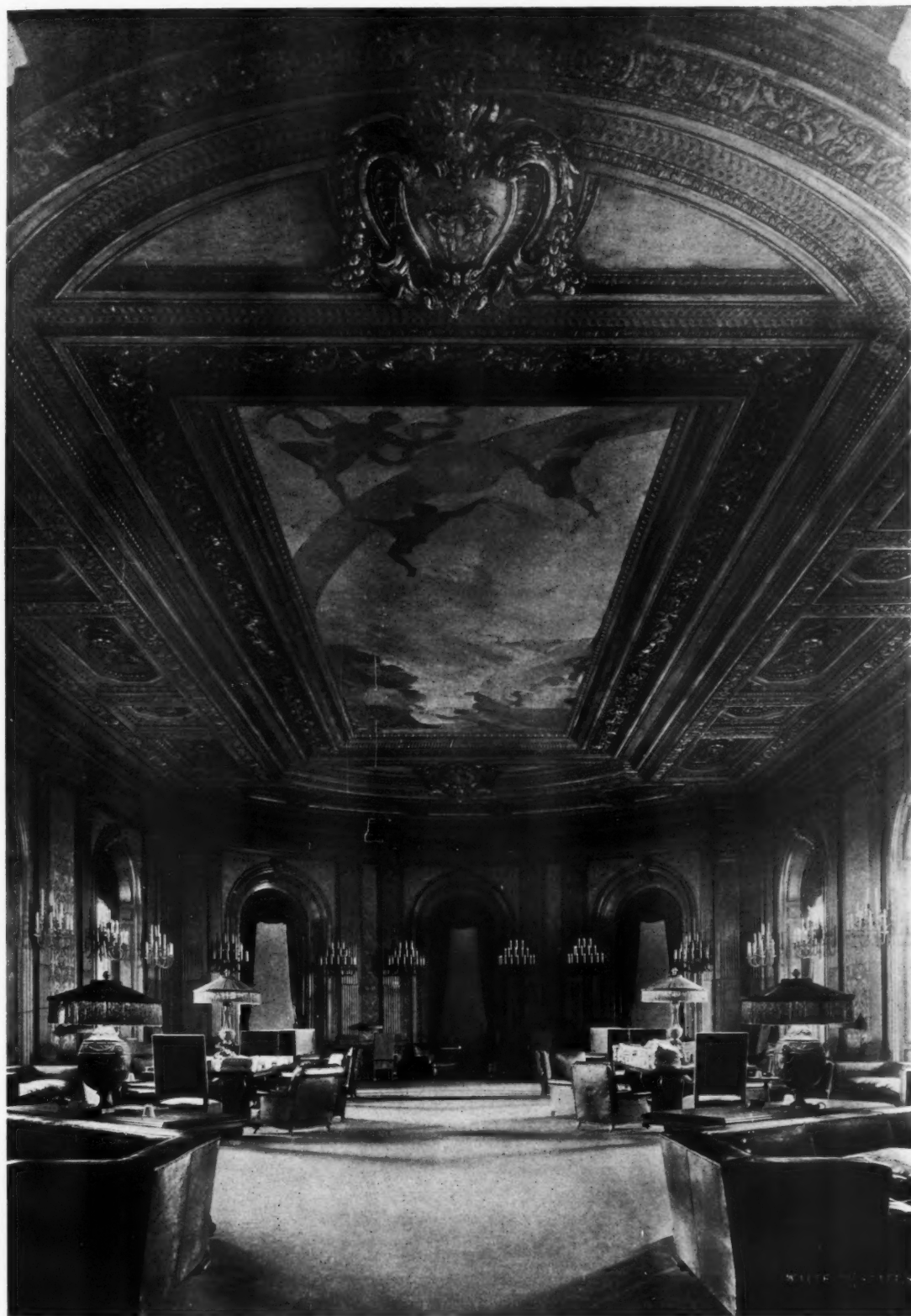
THE LOUNGING ROOM
