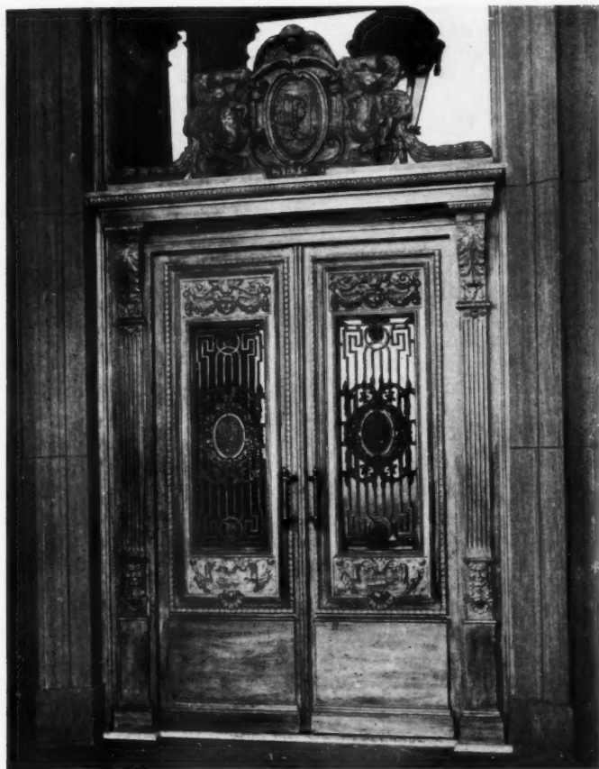
DETAIL OF ELEVATOR GATES
