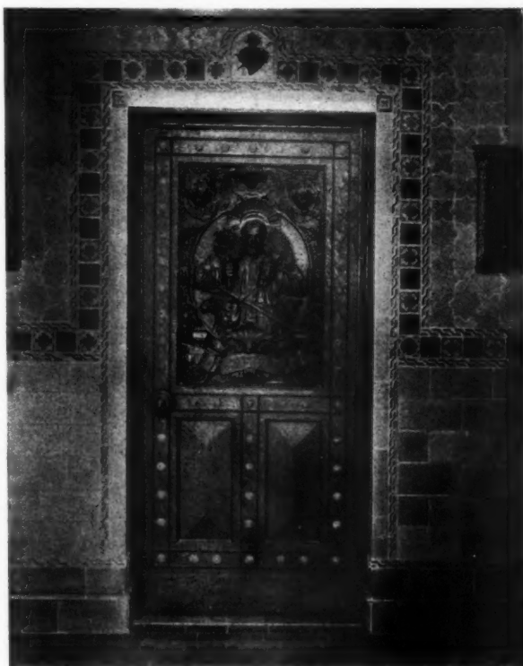
SACRISTY DOOR, ST. LAWRENCE CHURCH, ASHEVILLE, N. C. MR. R. S. SMITH, ARCHITECT
