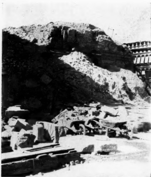
VIEW TAKEN A FEW DAYS AFTER THE COLLAPSE OF THE CAMPANILE IN 1902, SHOWING THE COMPLETE DAMAGE EFFECTED
