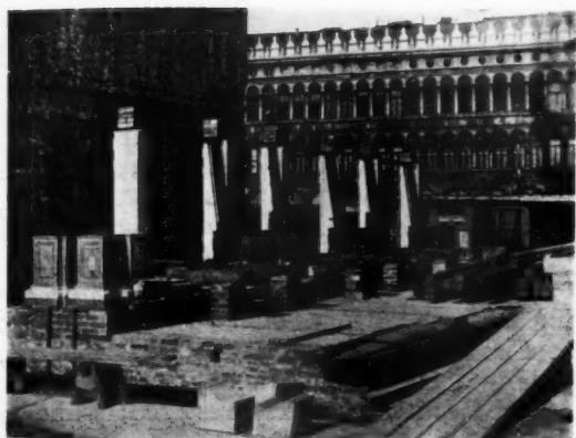
VIEW OF THE LOGGETTO DURING RECONSTRUCTION
