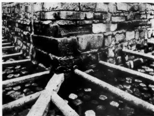
SHOWING THE WIDENING OF THE OLD FOUNDATION OF THE TOWER
