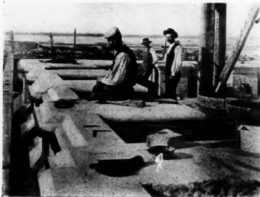
PARAPET OF THE BELL CHAMBER OR BELFRY
