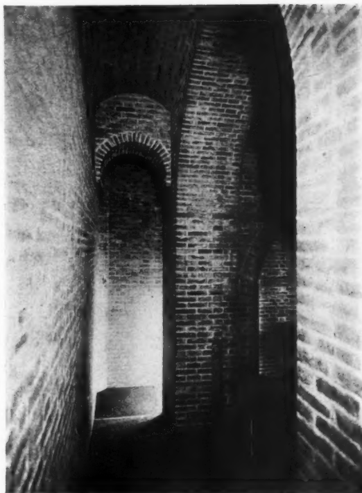
A VIEW IN THE INTERIOR OF THE NEW CAMPANILE, SHOWING THE SLOPING WAY
