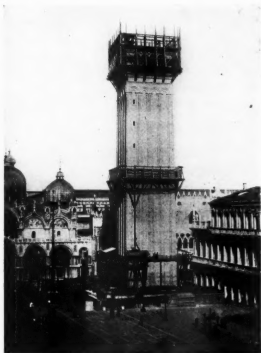
View copyrighted by Charles A. Braseler THE NEW CAMPANILE, SHOWING THE SLIDING PLATFORM IN PLACE OF THE USUAL SCAFFOLDING
