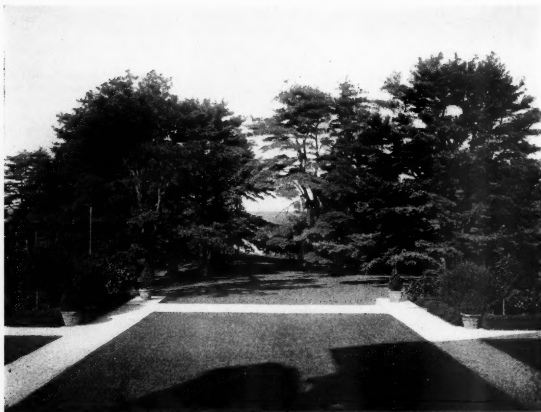
"SYLVANIA," BARRYTOWN, N. Y., MR. CHARLES A. PLATT, ARCHITECT
