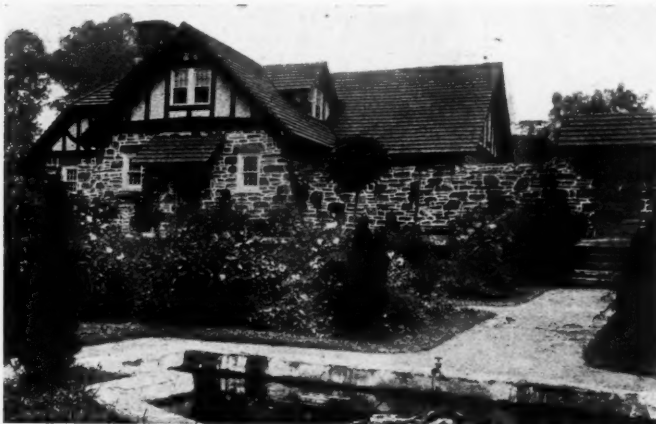
GARDEN AND GARAGE, ESTATE OF GRANVILLE H. LE MAISTRE, ESQ., MERION, PA.
