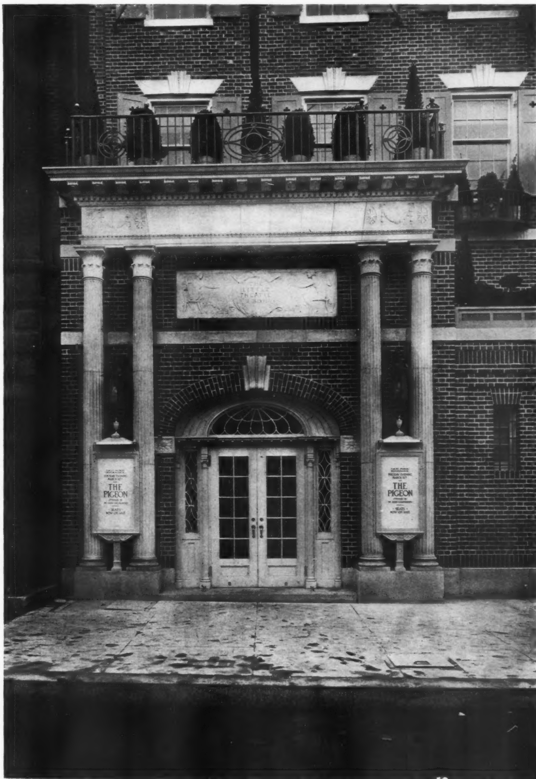
DETAIL OF ENTRANCE
