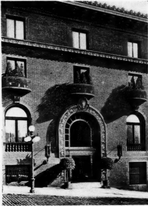
Detail of Entrance, The Bohemian Club, San Francisco, Cal. Messrs. L. P. Rixford & G. W. Vielham, Architects
