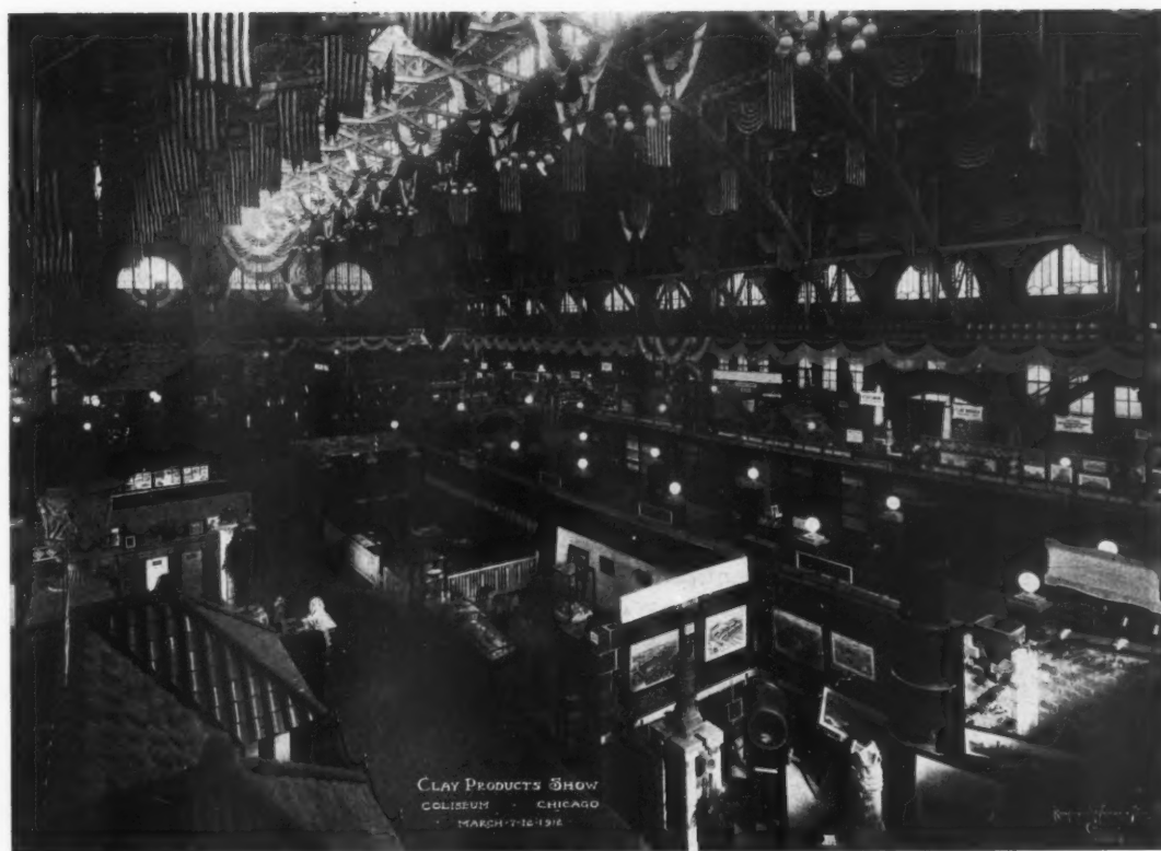
THE CLAY PRODUCTS EXPOSITION. VIEW IN COLISEUM BUILDING, CHICAGO
