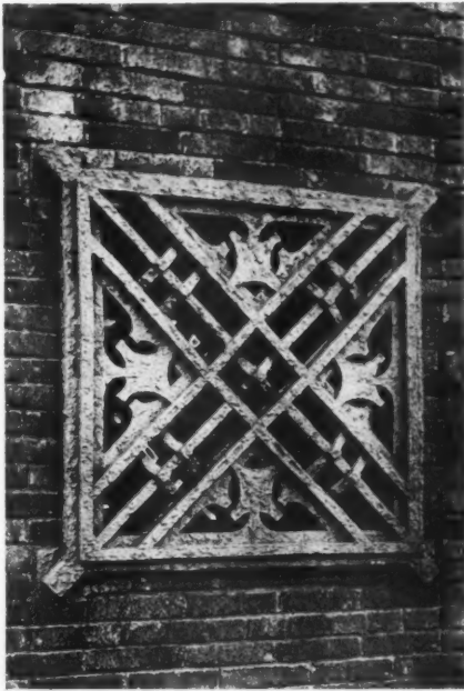
TERRA COTTA GRILLE OF CHIMNEY THE PEOPLES SAVINGS BANK, CEDAR RAPIDS, IOWA LOUIS H. SULLIVAN, ARCHITECT
