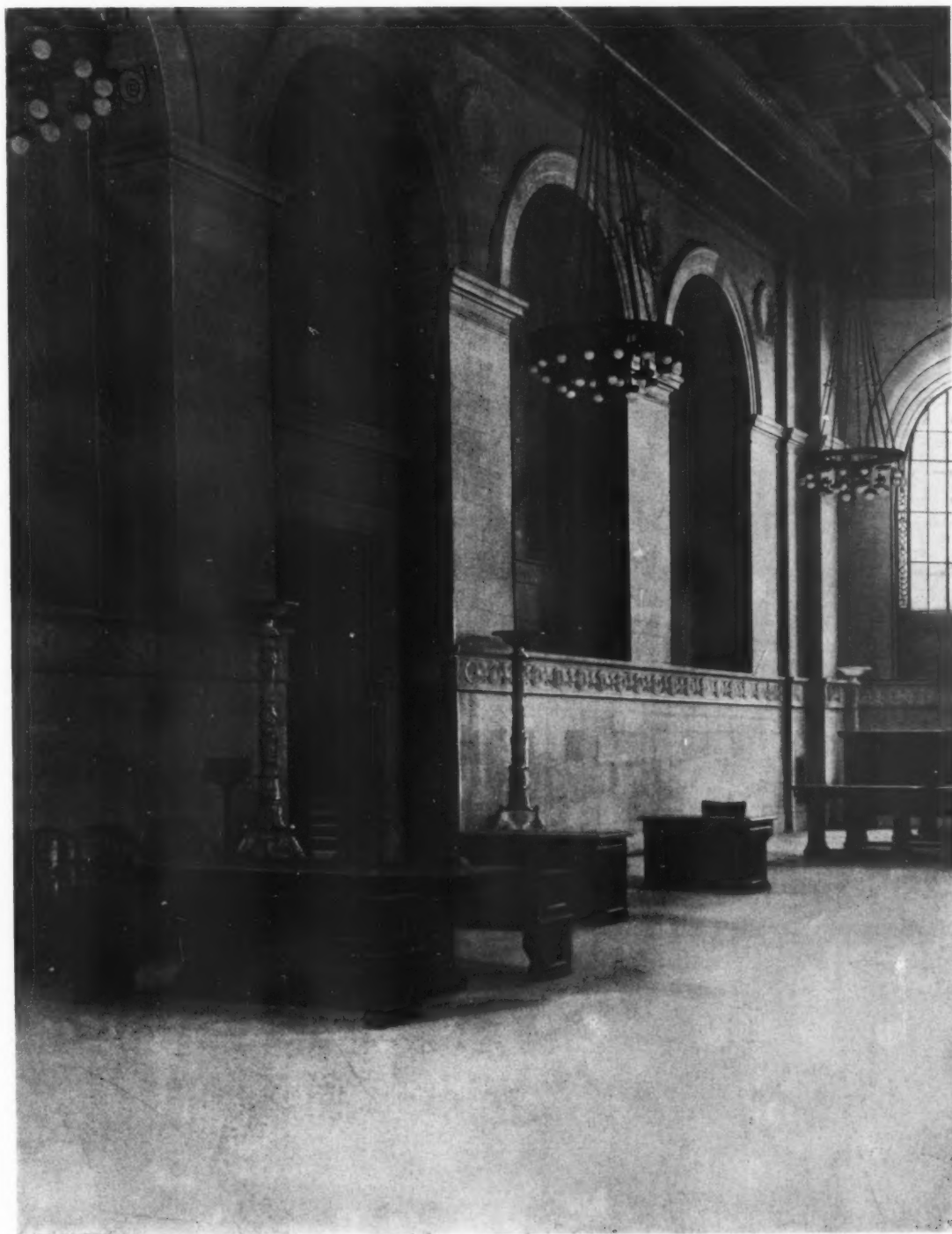
DELIVERY ROOM—DETAIL OF SOUTH WALL
