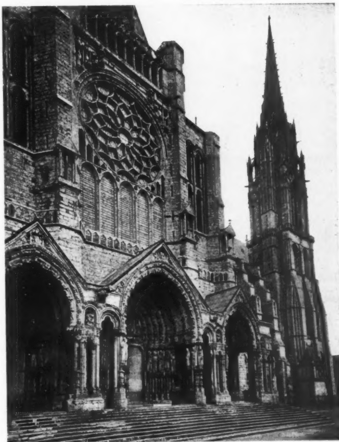
Exterior of the great rose window, north transept, Chartres Cathedral, showing the numerous horizontal bars.
