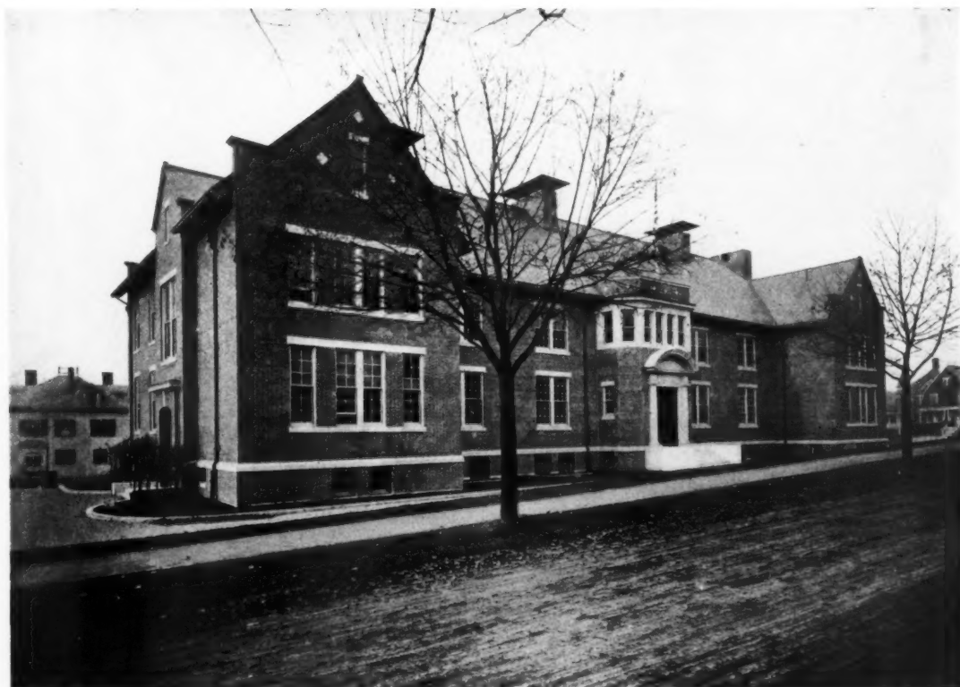
THE MICHAEL DRISCOLL SCHOOL, BROOKLINE, MASS. MESSRS. KILHAM & HOPKINS, ARCHITECTS
