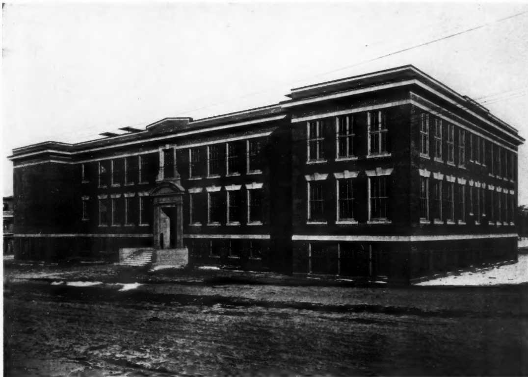
THE WILLIAMS SCHOOL, CHELSEA, MASS. MESSRS. KILHAM & HOPKINS, ARCHITECTS
