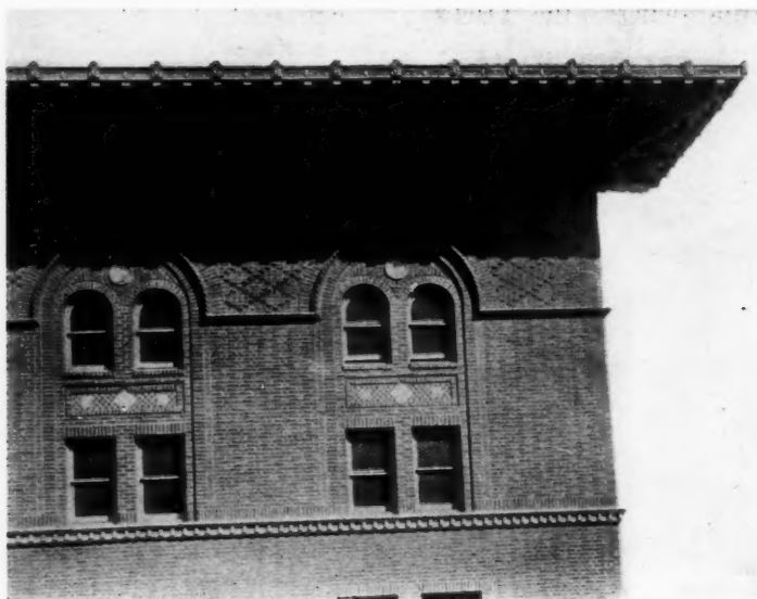
DETAIL OF UPPER STORIES, NORFOLK, VA., Y. M. C. A. BUILDING
