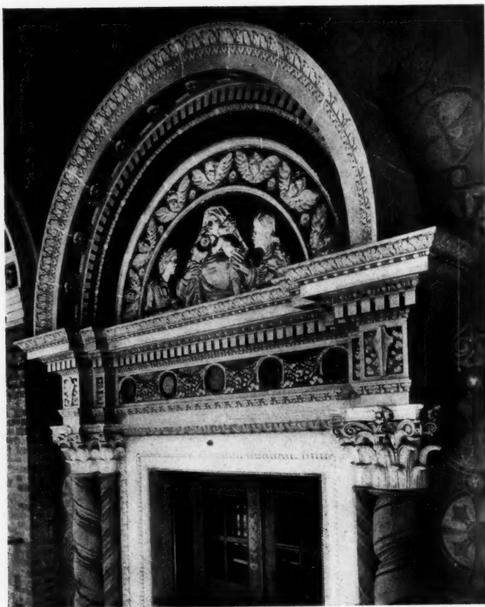
DETAIL OF ENTRANCE CHILDREN'S HOSPITAL, SAN FRANCISCO, CAL. MESSRS. BLISS & FAVILLE, ARCHITECTS
