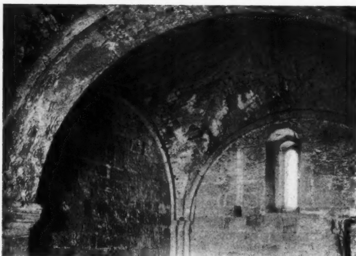
Fig. 3. The groined cross-vault in Italy, built without solid centering, on skeleton diagonals. Vault, in crypt, S. Maria del Solario, Brescia. Dating about 1120.
