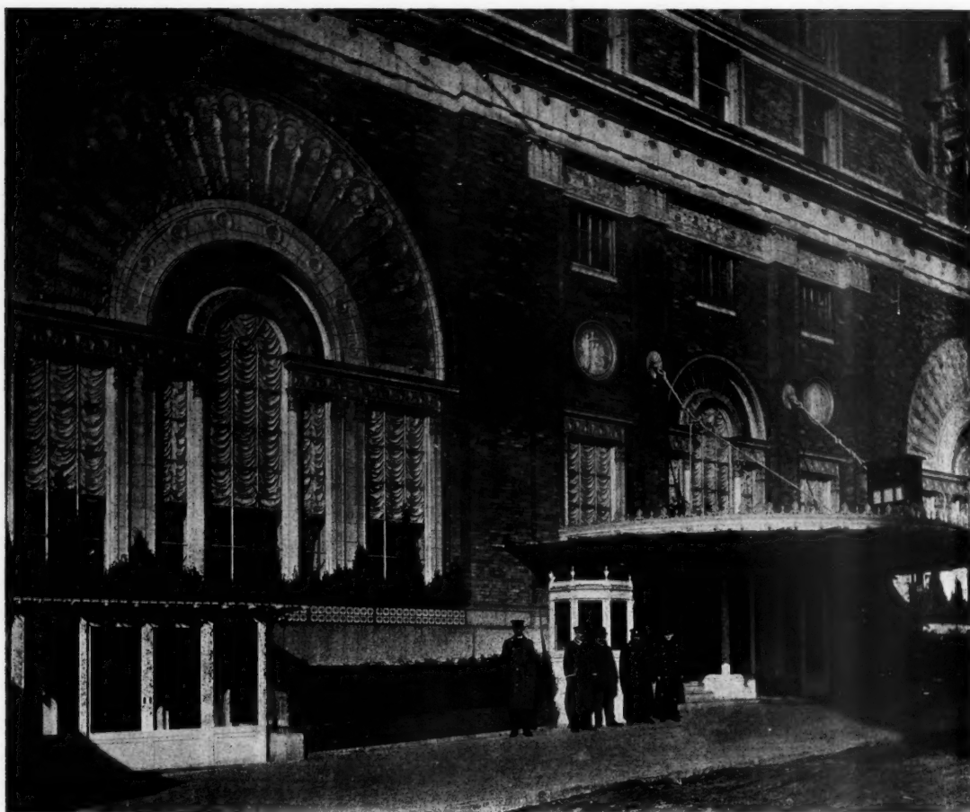
Main frontage, showing treatment of windows and introduction of terra-cotta relief. The ornament is low in relief and cream in tone. The walling is of semi-glazed brick, mottled, in shades of blue-grey and plum
