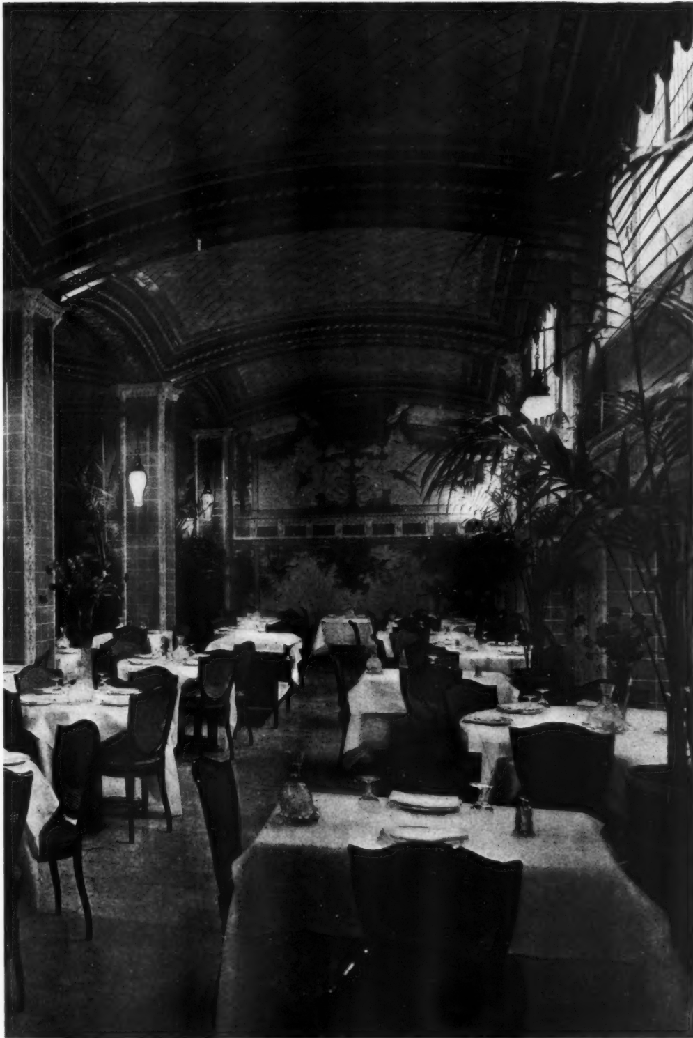
Another view in the Della Robbia room, showing the general spread of vaulting and treatments of wall surfaces. Note the frank acceptance of the radiators and skillful handling of festooning. The blues of the tile enter freely into the painting.
