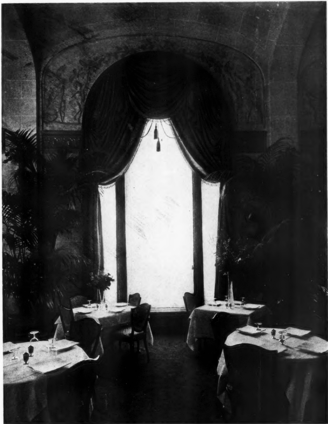
View showing treatment of main windows to the dining room portion of the central hall. Spandrels, pilasters and vaulting are of plaster in imitation of Caen stone.
