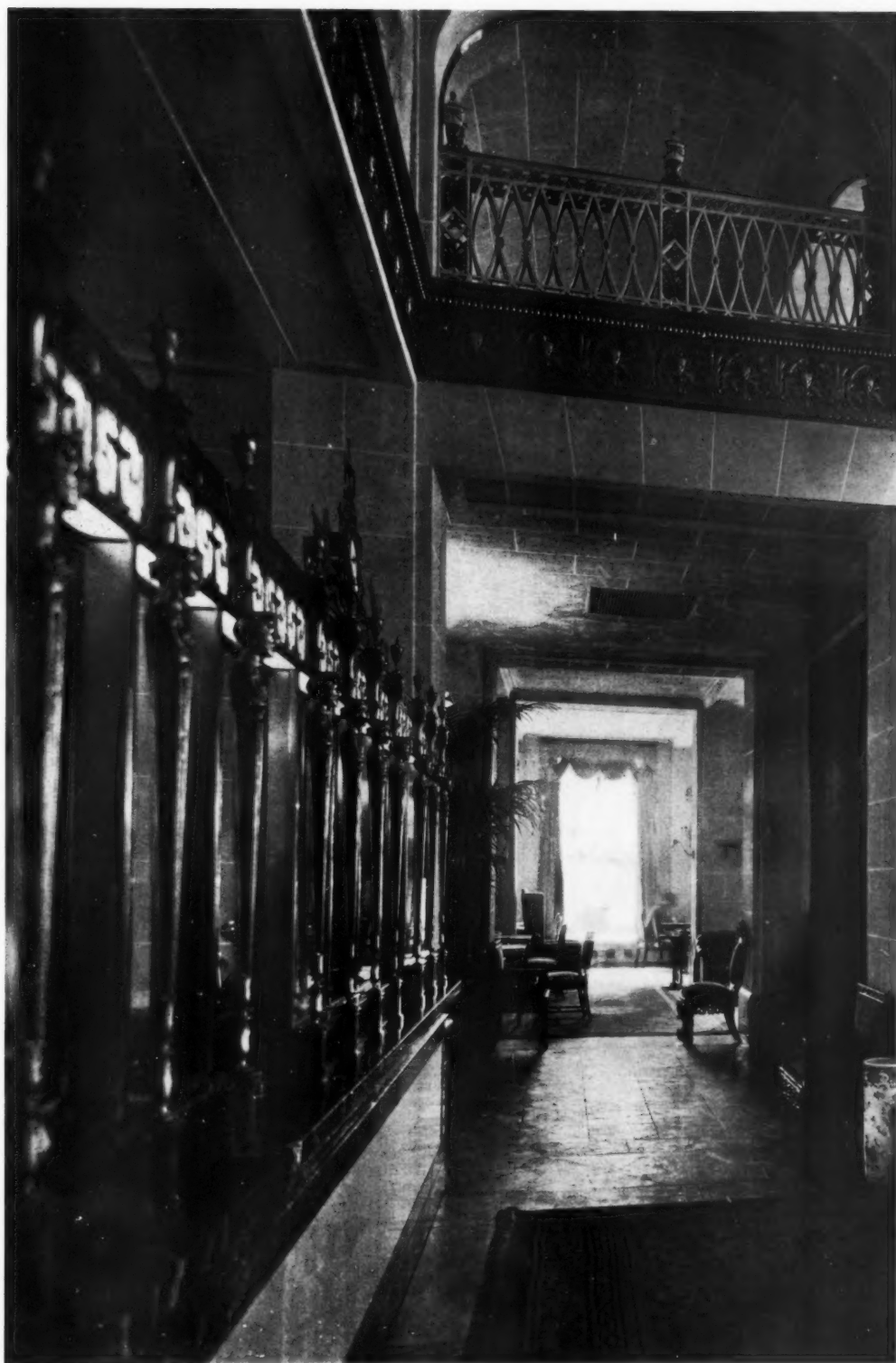
Main office, showing brass screen, detail of ceiling under balcony and vaulting to central hall. The flooring is of Numidian Marble
