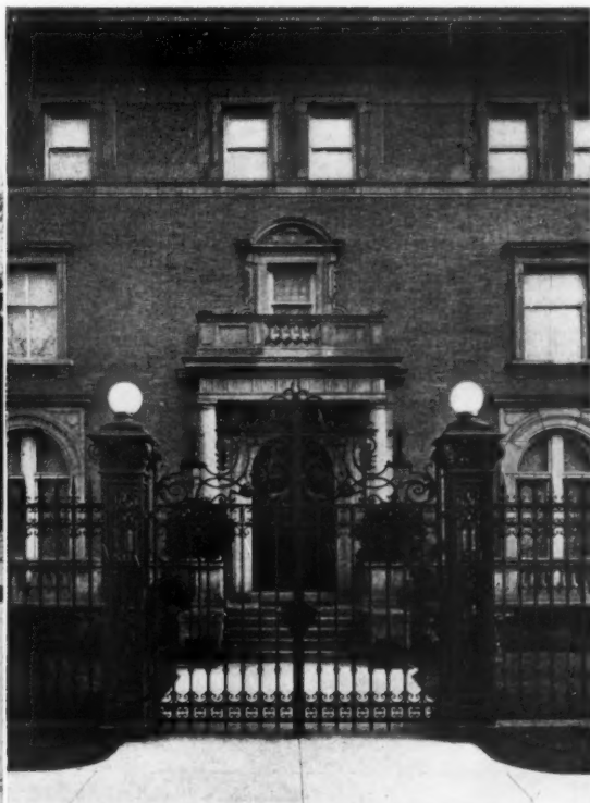
DETAIL OF MRS. CHRISTIAN STENGEL'S RESIDENCE, NEWARK, N. J. MR. WARRINGTON G. LAWRENCE, ARCHITECT
