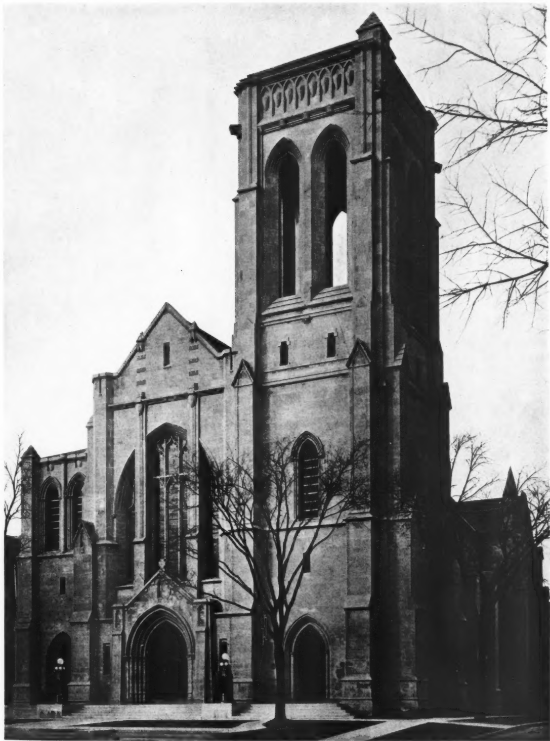
VIEW FROM NORTHEAST
