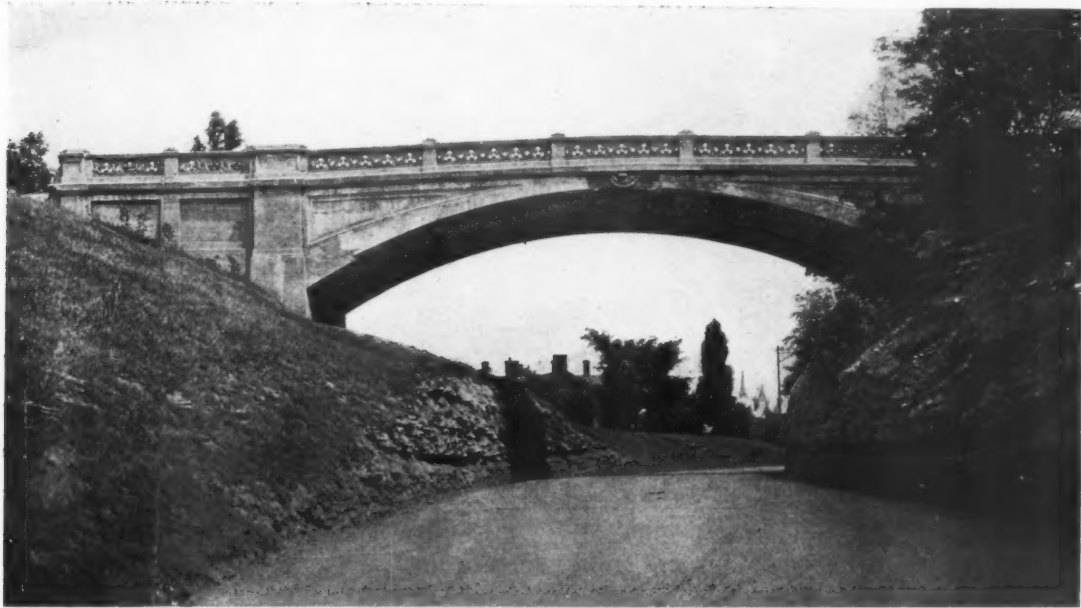
CONCRETE-STEEL ARCH BRIDGE, EDEN PARK, CINCINNATI, O.
