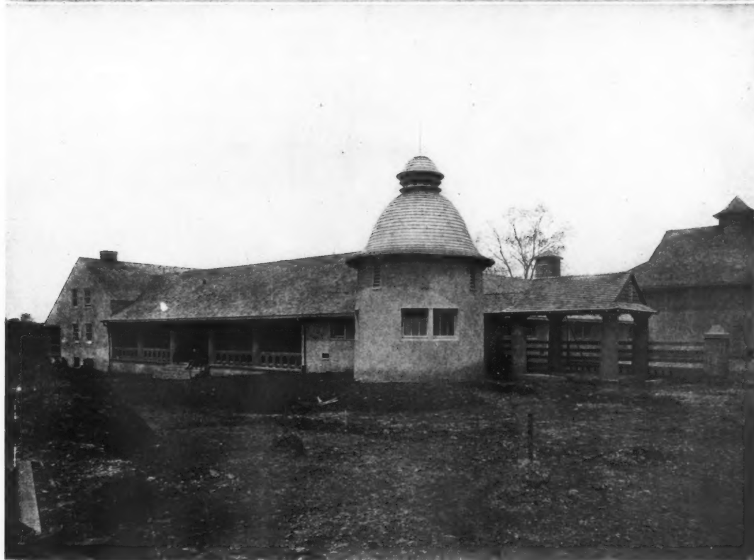
ABOVE, A WAGON AND MACHINERY SHED OF REINFORCED CONCRETE, PABST STOCK FARM AT OCONOMOWOC, WIS., MESSRS. FERNEKES & CRAMER, ARCHITECTS BELOW, FARM LABORER'S COTTAGES AND BARN
