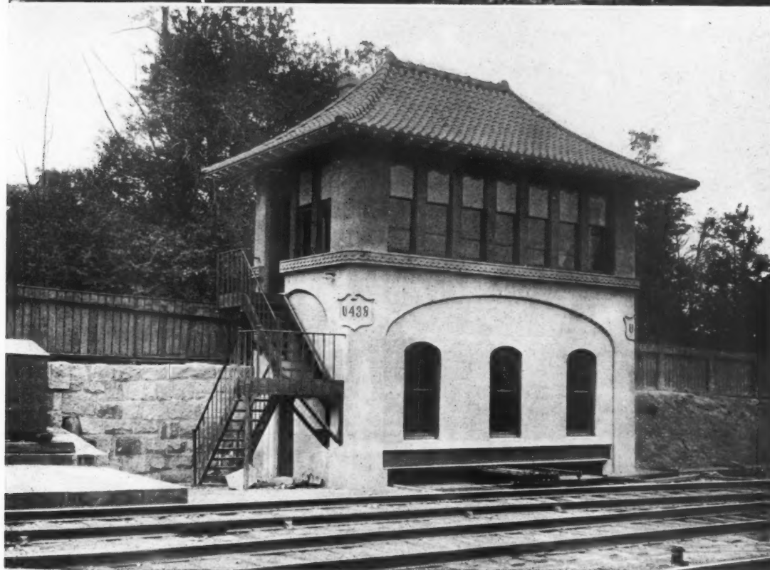
ABOVE, A CONCRETE PUBLIC COMFORT STATION, SHOWING THE RESULTS OF GOOD FORM CONSTRUCTION AND CAREFUL MIXING AND PLACING. BELOW, A SOLID CONCRETE SWITCH TOWER ON NEW YORK, NEW HAVEN & HARTFORD RAILWAY AT SAVIN HILL, MASS.
