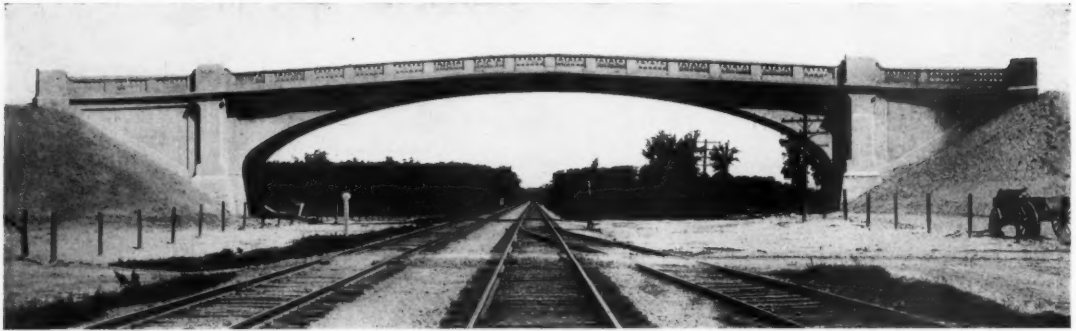
A CONCRETE BRIDGE SHOWING GOOD ARCHITECTURAL TREATMENT
