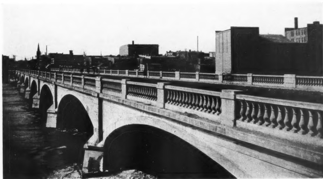
A GOOD EXAMPLE OF MODERN CONCRETE BRIDGE CONSTRUCTION
