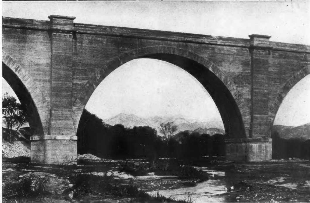
ABOVE, PORTAL OF A TUNNEL, SHOWING THE POSSIBILITIES OF CONCRETE IN RAILWAY CONSTRUCTION. BELOW, SECTION OF CONCRETE BRIDGE ON SALT LAKE RAILWAY, NEAR RIVERSIDE, CAL.
