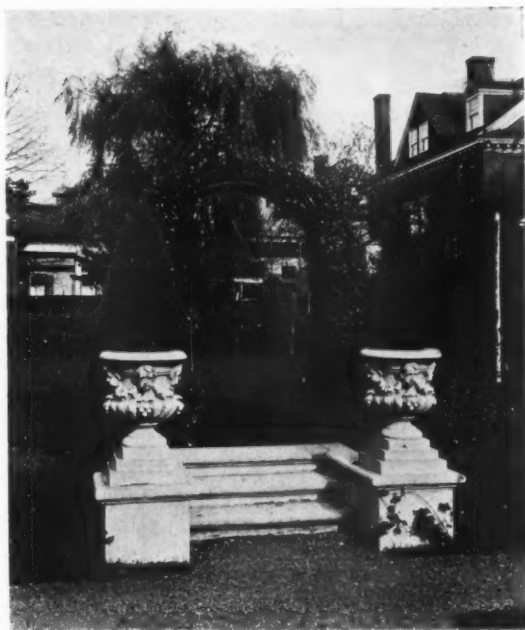
A WELL-EXECUTED CONCRETE GARDEN DETAIL
