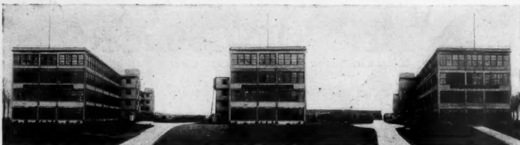
FRONT VIEW OF CHALMERS MOTOR CO. PLANT, DETROIT, MICH. ALBERT KAHN, Architect
