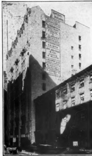
Spero Building, New York City Raydiant Sidewalk Lights Installed Robert D. Kohn, Architect C. A. Cowen, General Contractor
