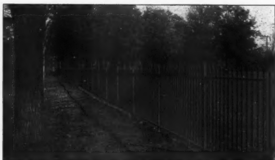
There are 1800 feet of this 5-foot iron railing around the Plainfield Union Water Co. at Plainfield, N. J.
