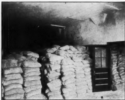
Warehouse of the Powers Transfer & Storage Company, Minneapolis, Minn. The floors were designed for a 200-lb. load and were tested to 400 lbs.
