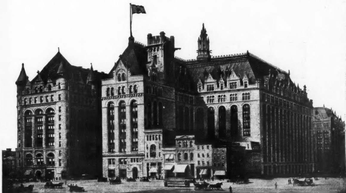
PRUDENTIAL BUILDING, NEWARK, N. J. Circuits controlled by G. E. Office Building Switchboard.
