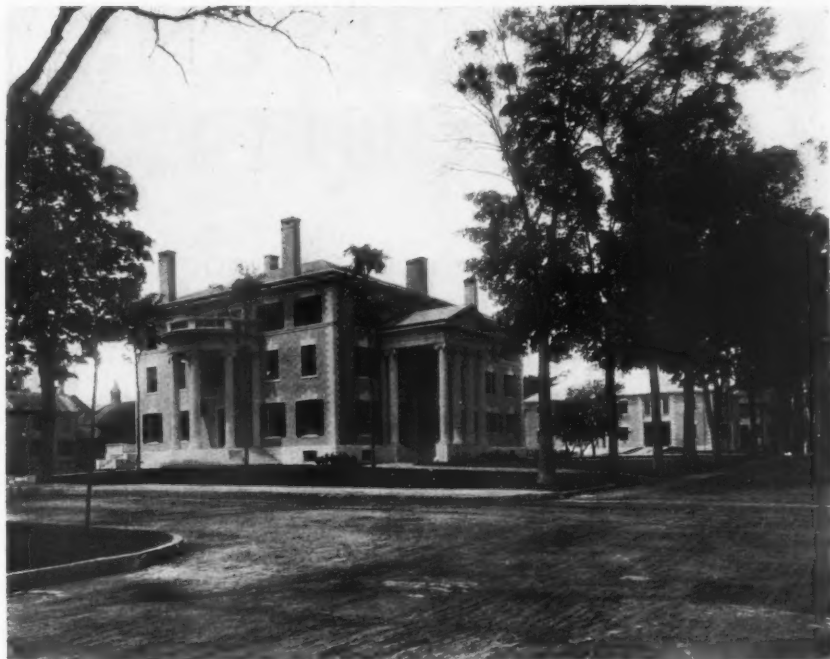
Residence of Ex-Governor John F. Hill, Augusta, Me. Equipped with Automatic Refrigerating Plant Messrs. John Calvin Stevens and John Howard Stevens, Architects, Portland, Maine.
