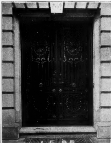
ENTRANCE DOORS, JAMES B. CLEWS' RESIDENCE.
