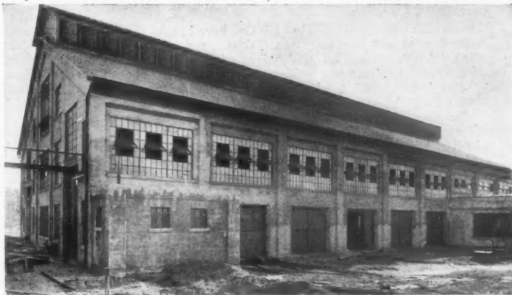
Forge Shop, Billings and Spencer Co. Messrs. Ford, Buck & Sheldon, Architects and Engineers
