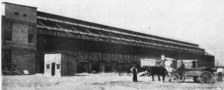
Forge Shop, Packard Motor Car Co., Detroit, Mich. Mr. Albert Kahn, Architect; Mr. Ernest Wilby, Associate
