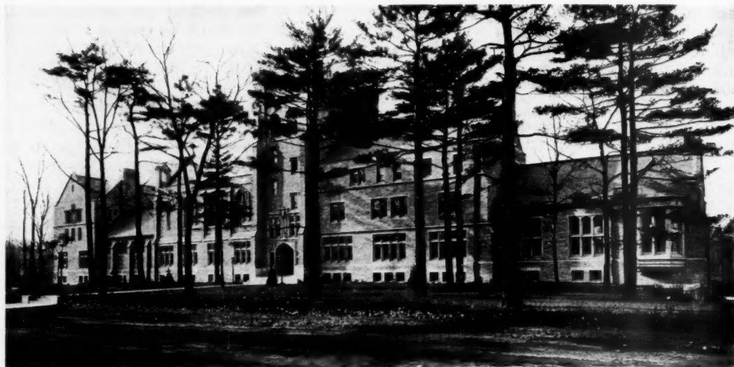
VIEW FROM NORTH EAST
