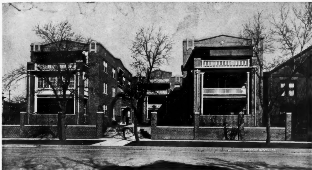
SORRENTO APARTMENTS, DENVER, COLO.
